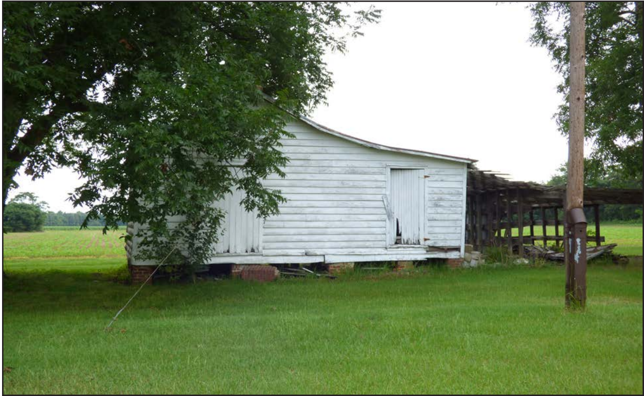
Photo 143. NS1493, agricultural outbuildings, facing north.
