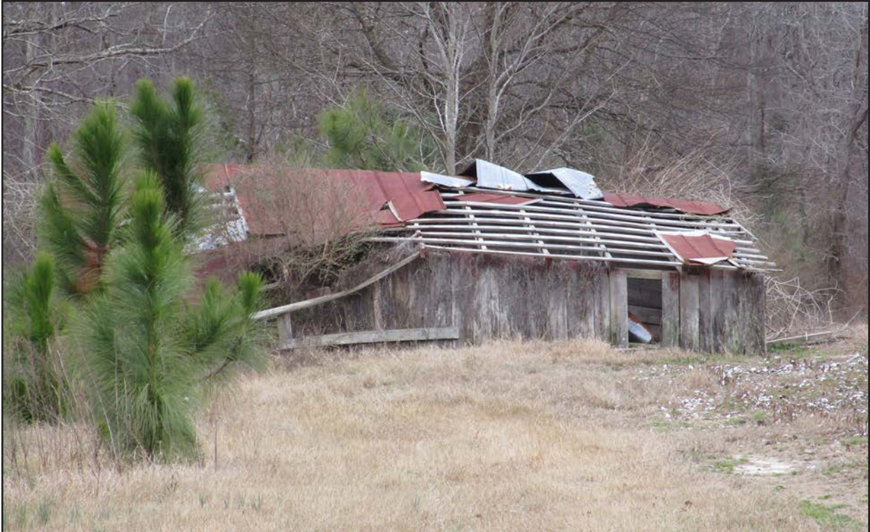
Photo 52. HX1581, storage structure, facing south.
