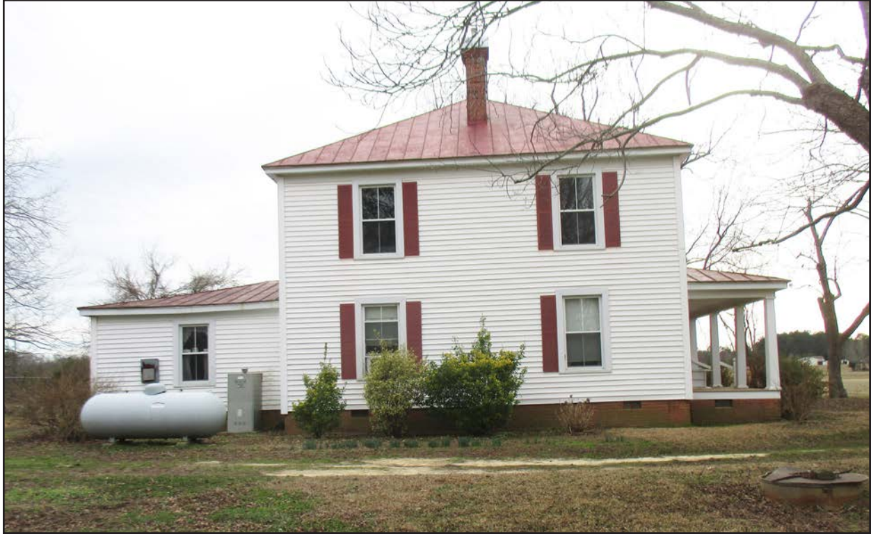
Photo 127. NS0650, house, facing south.
