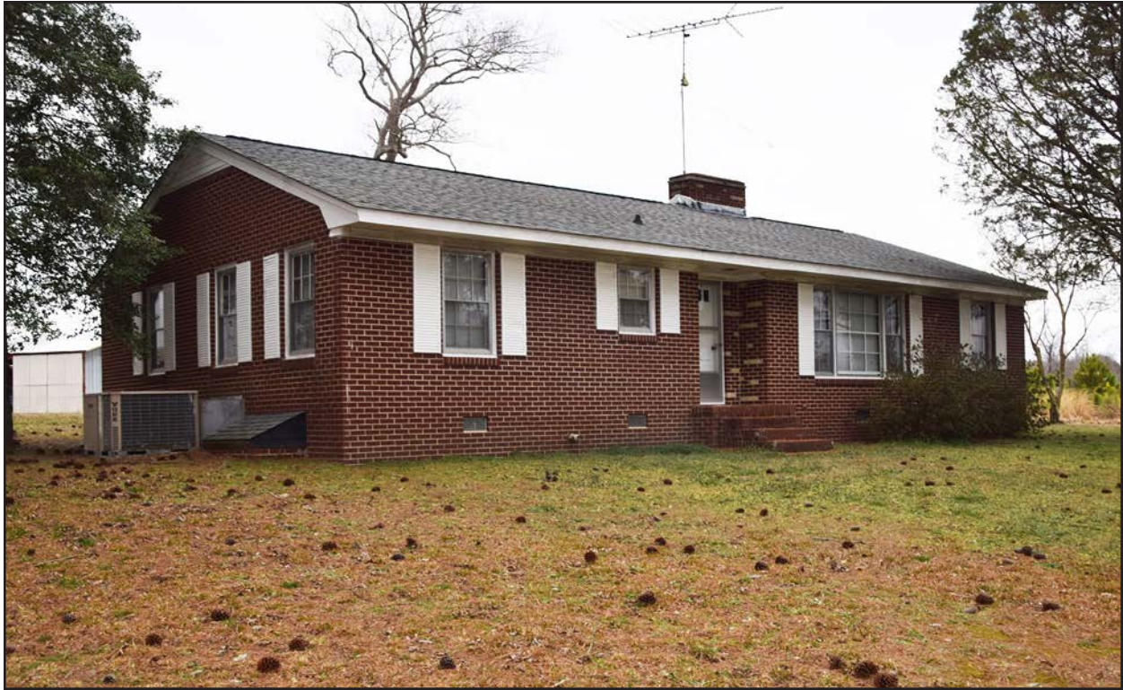
Photo 43. HX1581, facing north-northwest.
