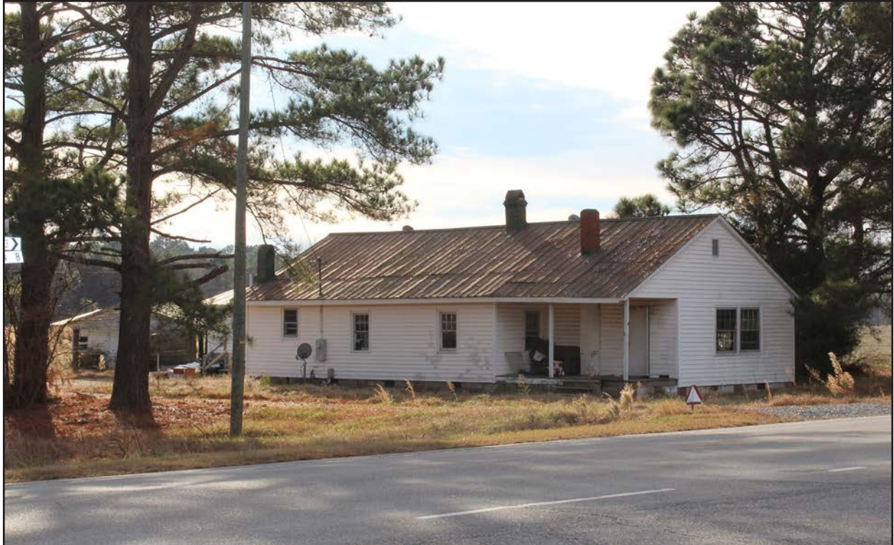
Photo 78. JT1864, house, facing southwest.
