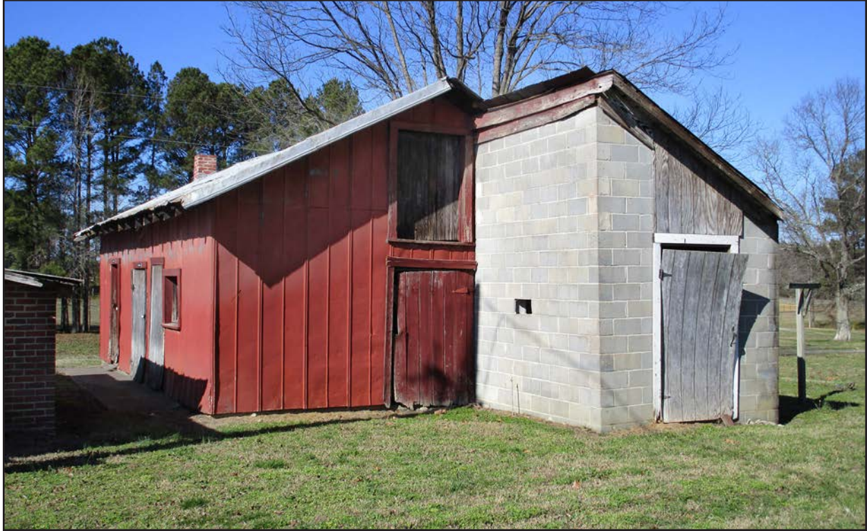
Photo 23. HX0021, wash room/laundry, shed roof addition, facing north-northwest.
