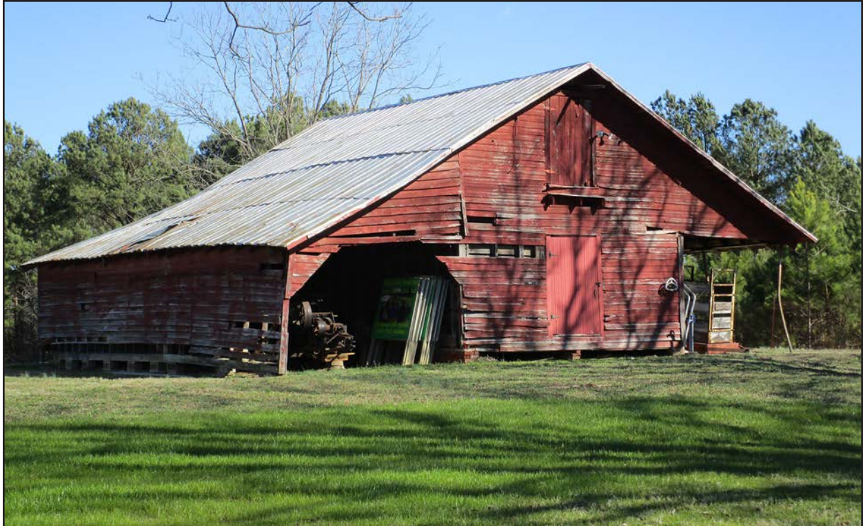
Photo 14. HX0021, corn and equipment barn, facing east-northeast.
