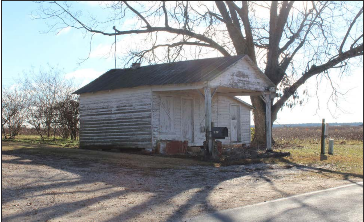
Photo 32. HX0227, rear accessory structure, facing southeast.
