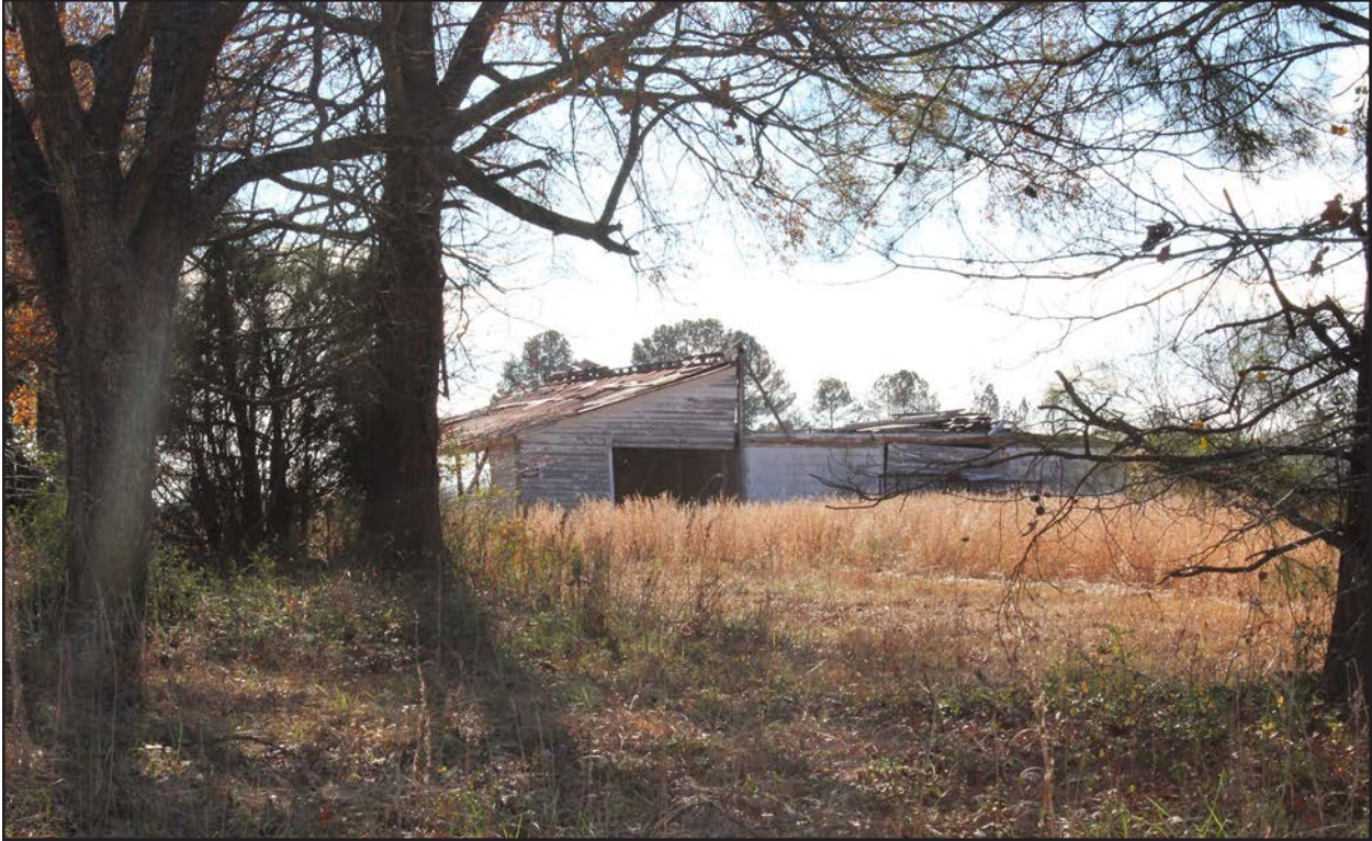
Photo 89. JT1919, accessory structure, facing south-southeast.
