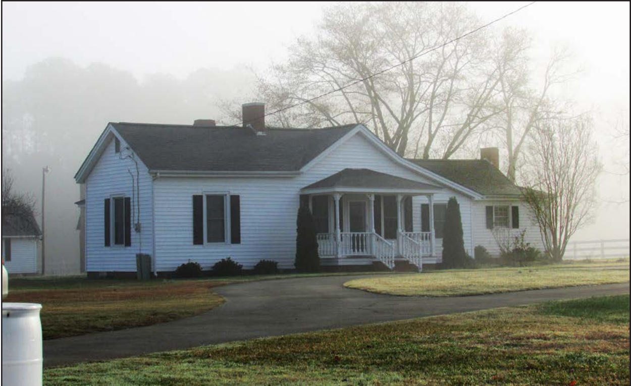
Photo 90. JT1920, facing east-southeast. Dove
