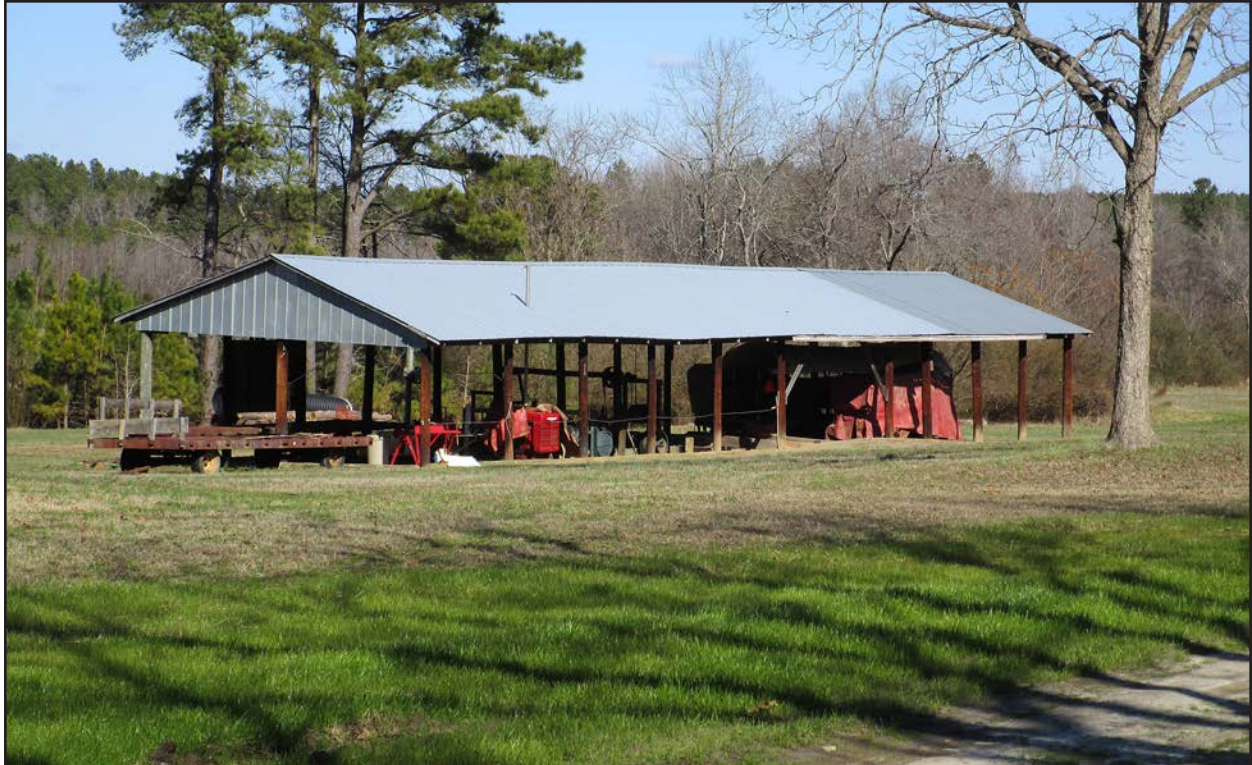
Photo 12. HX0021, equipment shed, facing north-northeast.
