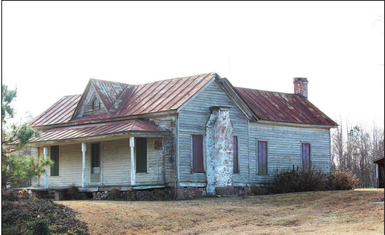
Photo 180. WL2012, facing southwest.
