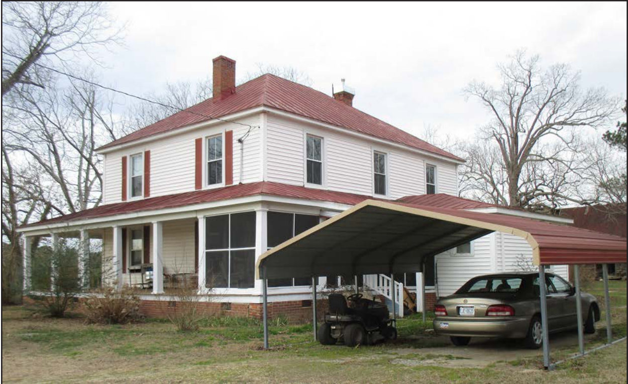
Photo 136. NS0650, carport, facing northwest.
