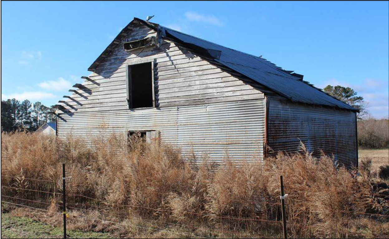
Photo 38. HX0229, facing southwest.
