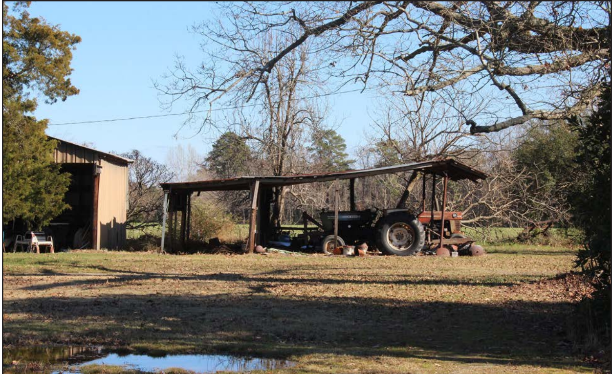
Photo 68. JT0957, pole shelter, facing east.
