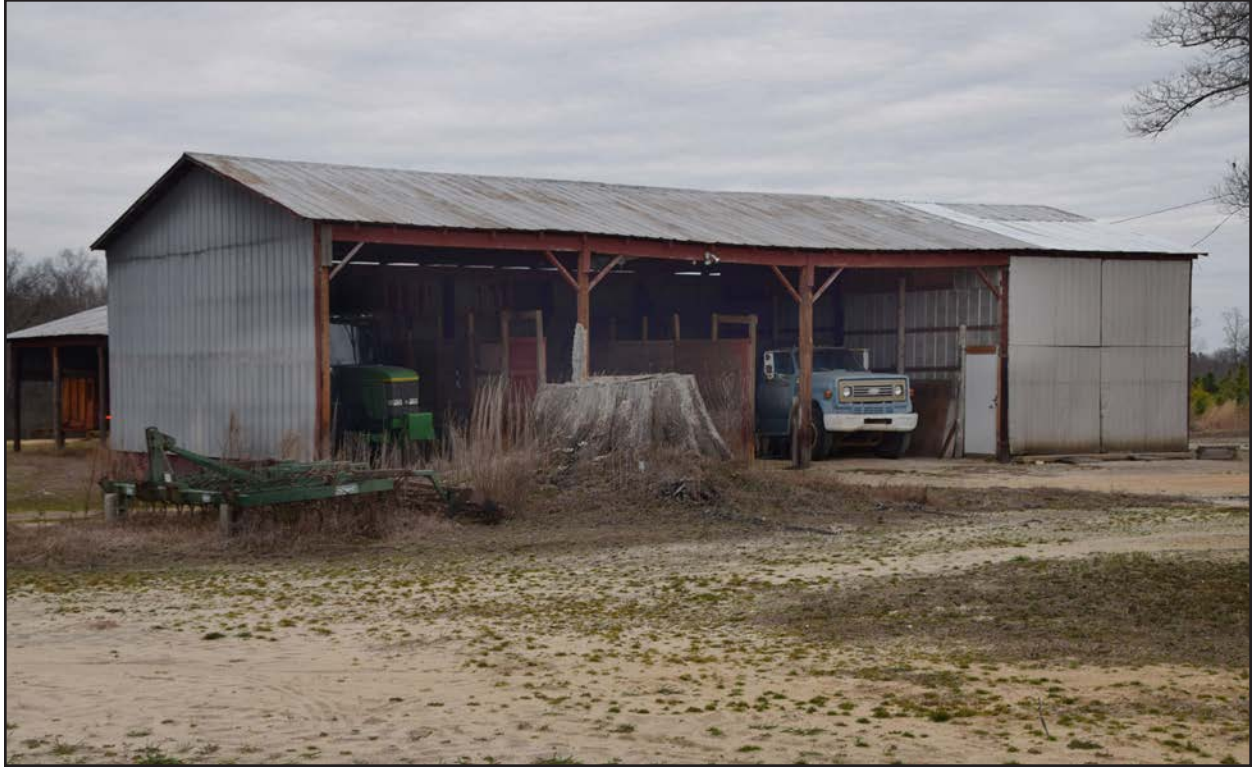
Photo 47. HX1581, garage, facing northeast.
