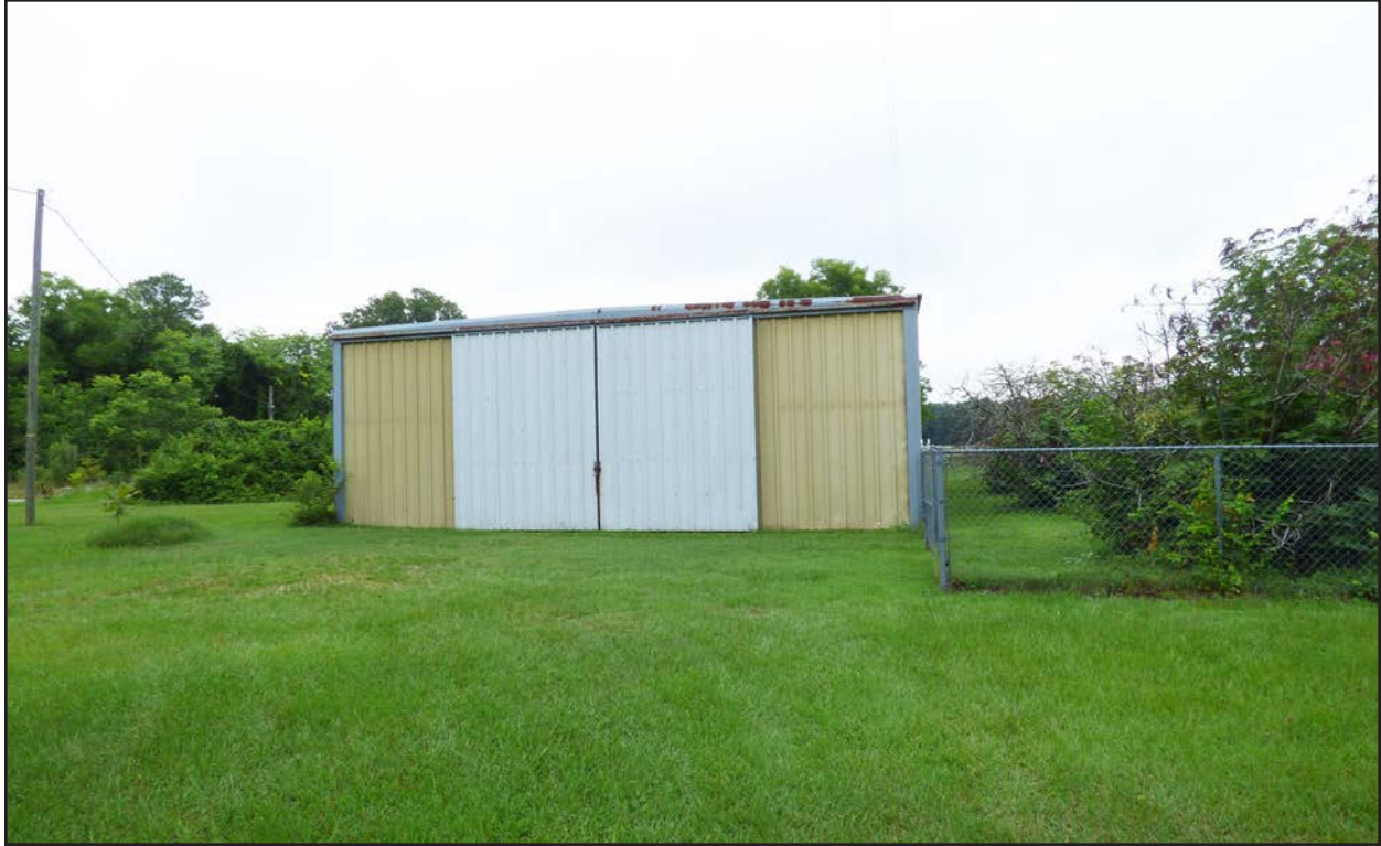
Photo 147. NS1493, metal workshop building, facing south.
