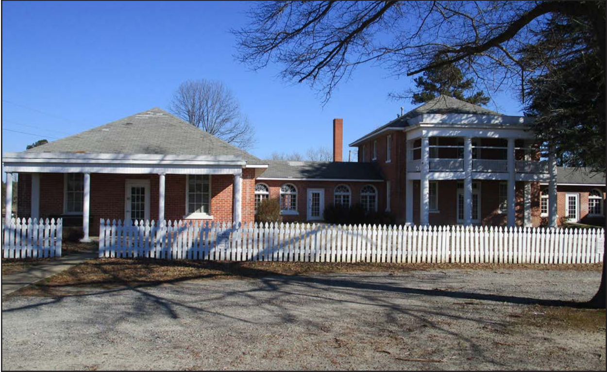
Photo 7. HX0021, facing northeast.
