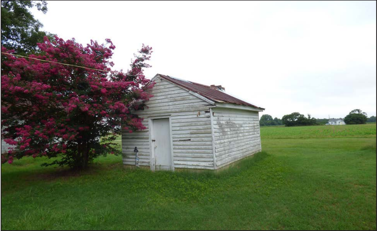
Photo 141. NS1493, agricultural outbuilding, facing northwest.
