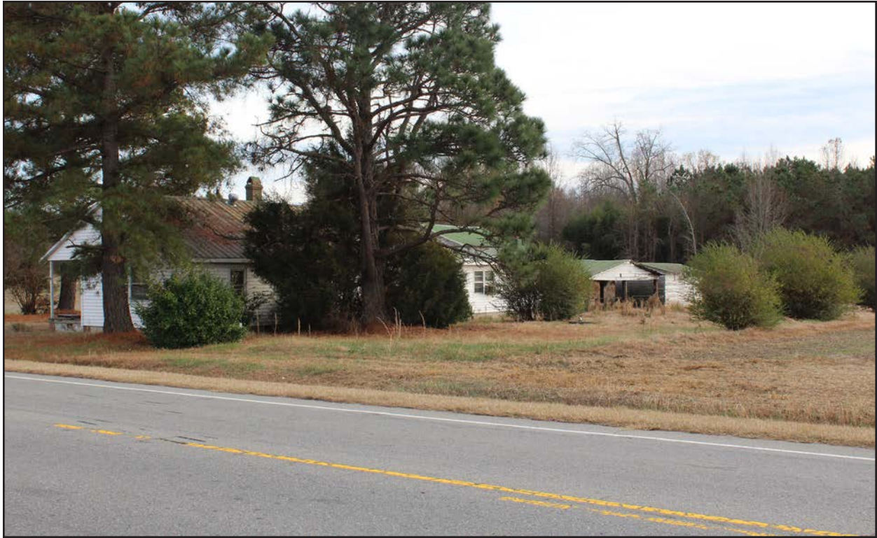
Photo 79. JT1864, house with rear wings, facing southeast.
