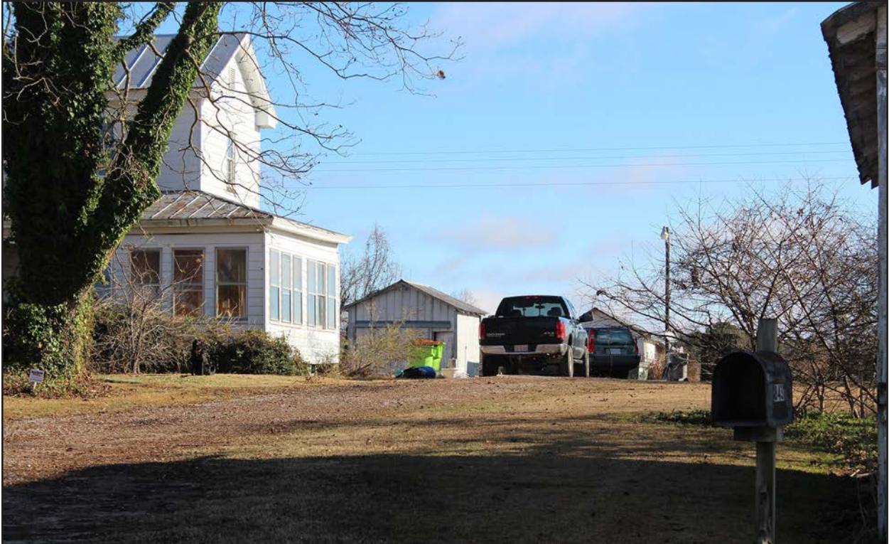
Photo 30. HX0227, rear accessory structure, facing east.
