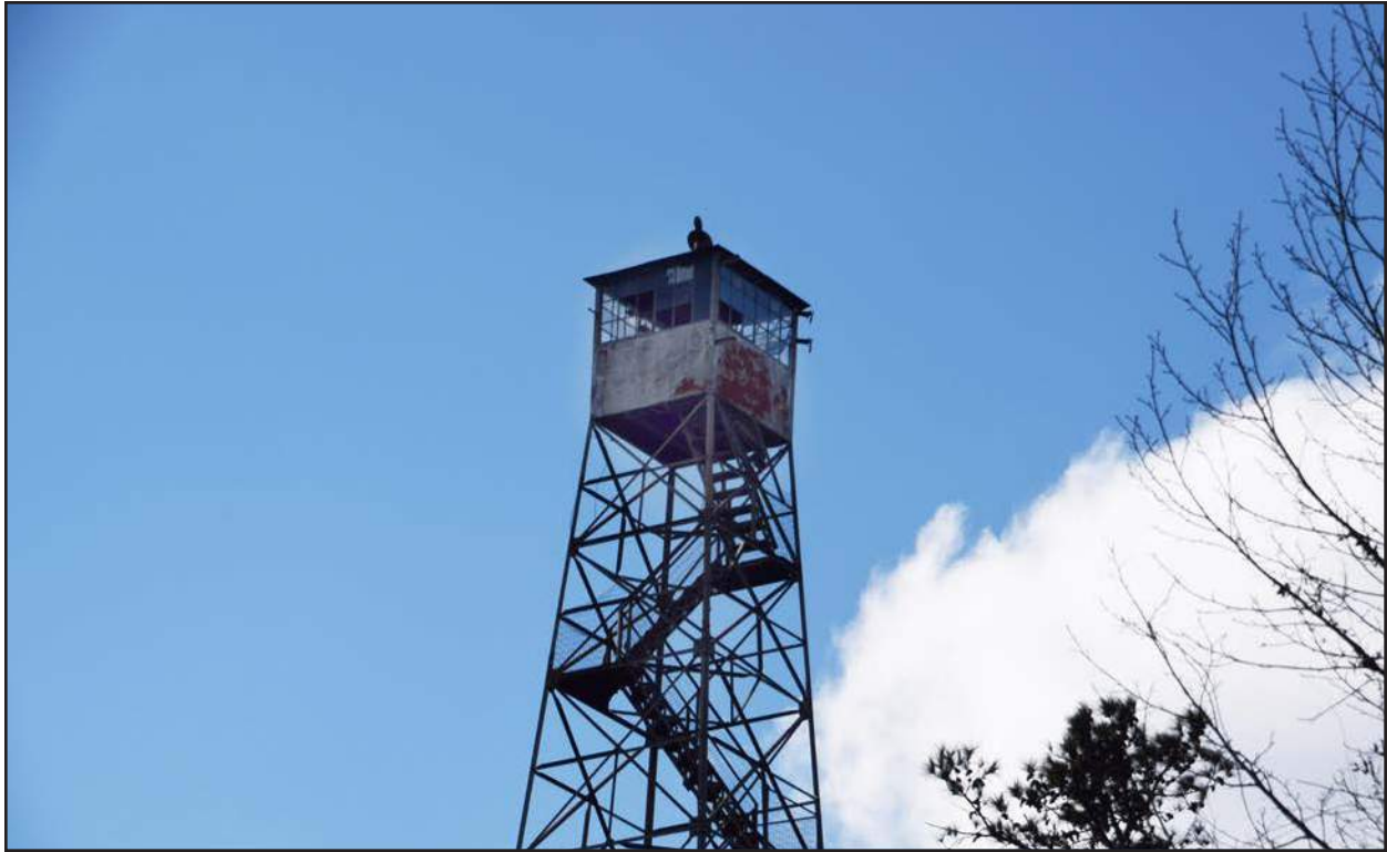
Photo 75. JT1860 (Smithfield Fire Lookout Tower), fire tower observation box, facing west-southwest.
