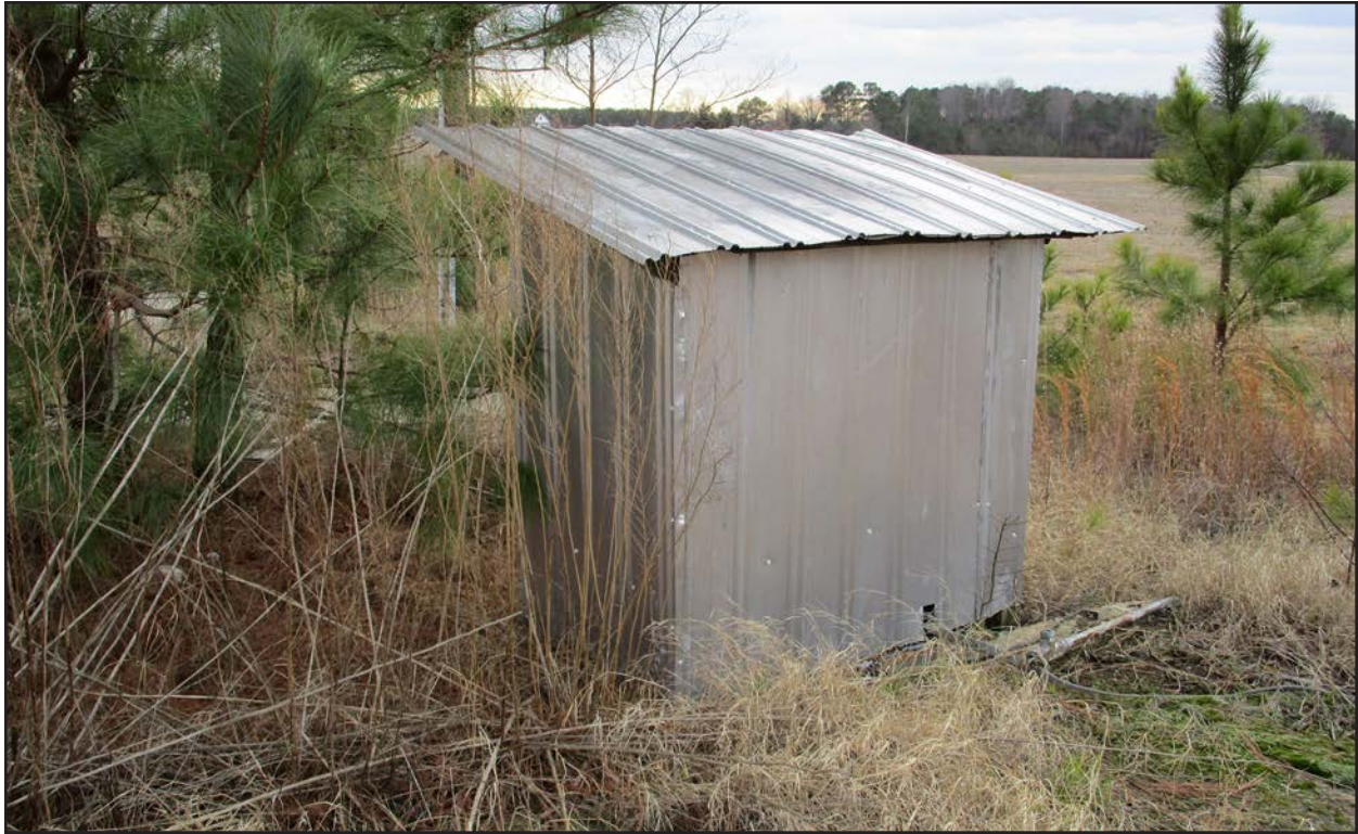
Photo 157. NS1508, small shed, facing southeast.
