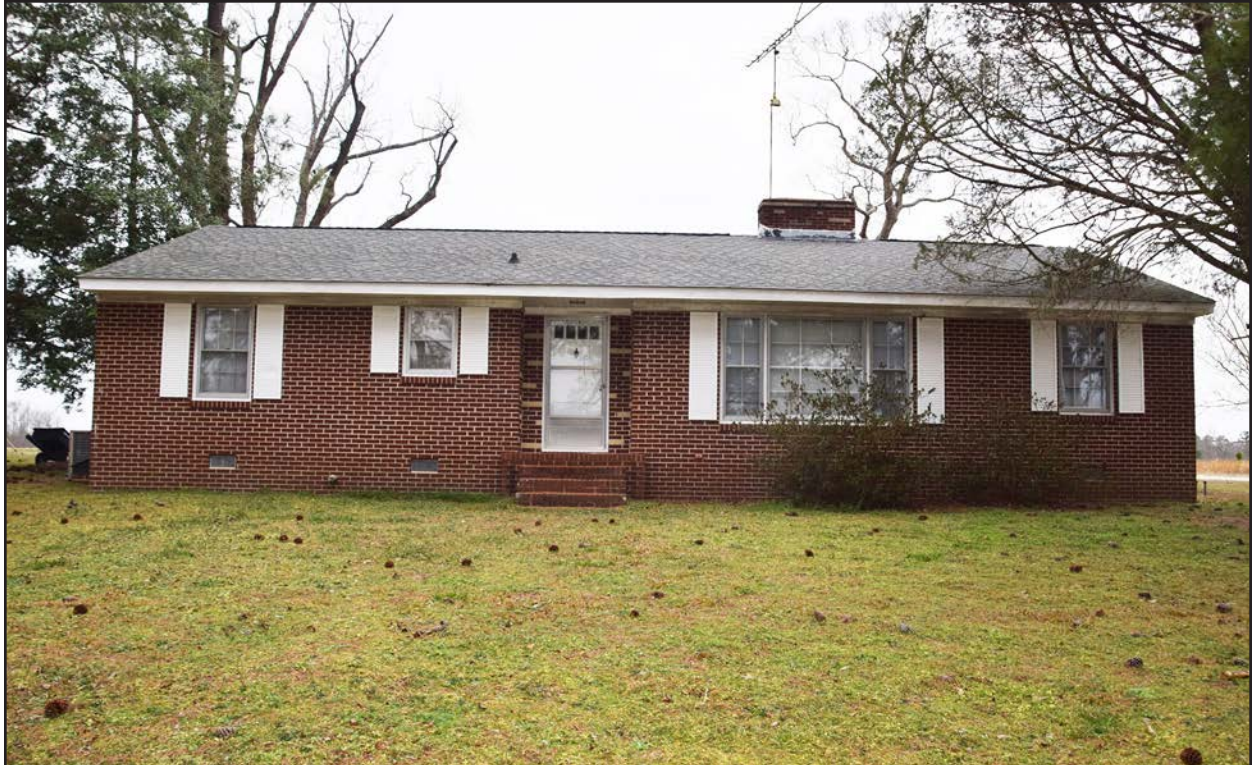
Photo 44. HX1581, facing north-northwest.
