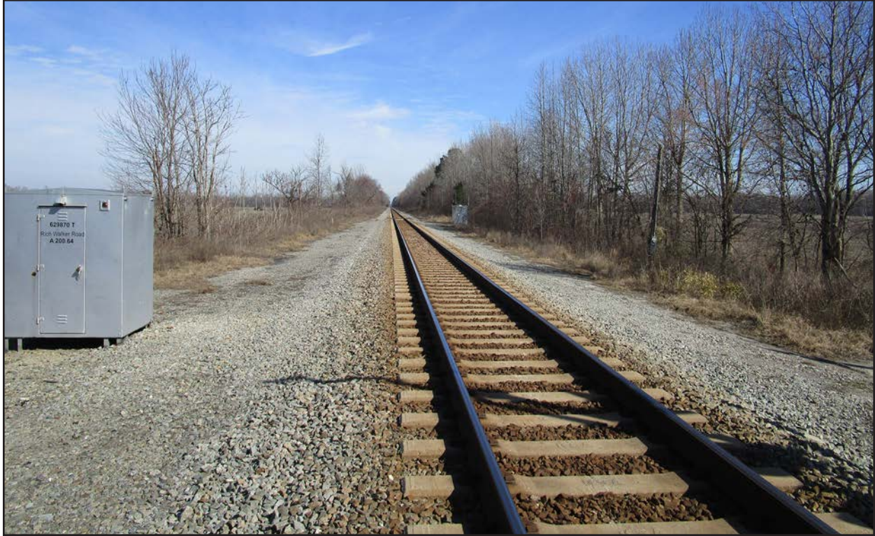
Photo 1. CD1450 (Fayetteville Cutoff), facing west.
