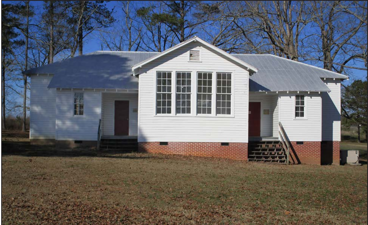
Photo 42. HX1566 (Allen Grove Rosenwald School), facing northwest.
