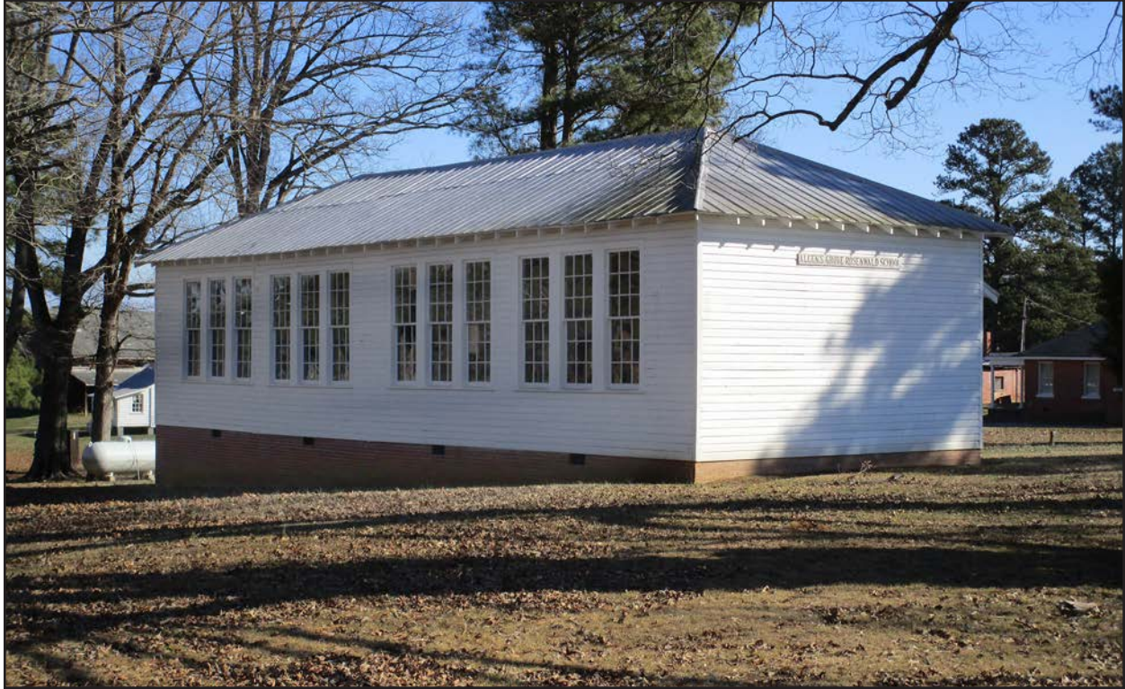
Photo 41. HX1556 (Allen Grove Rosenwald School), facing east.
