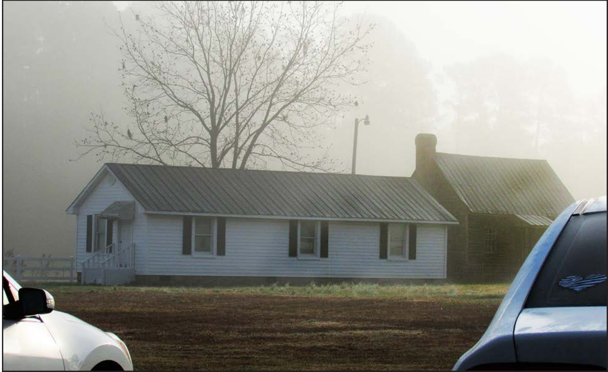
Photo 93. JT1920, accessory structure 2, facing southeast.
