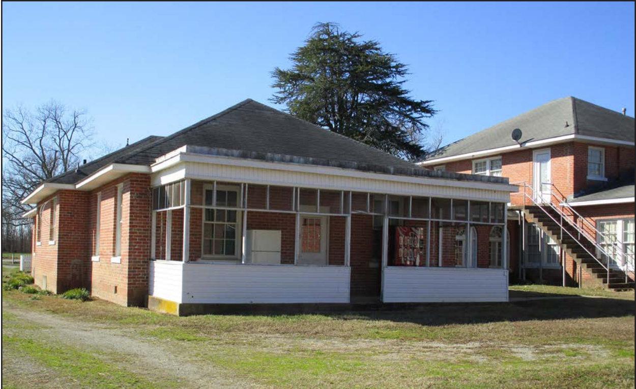
Photo 8. HX0021, facing southwest.
