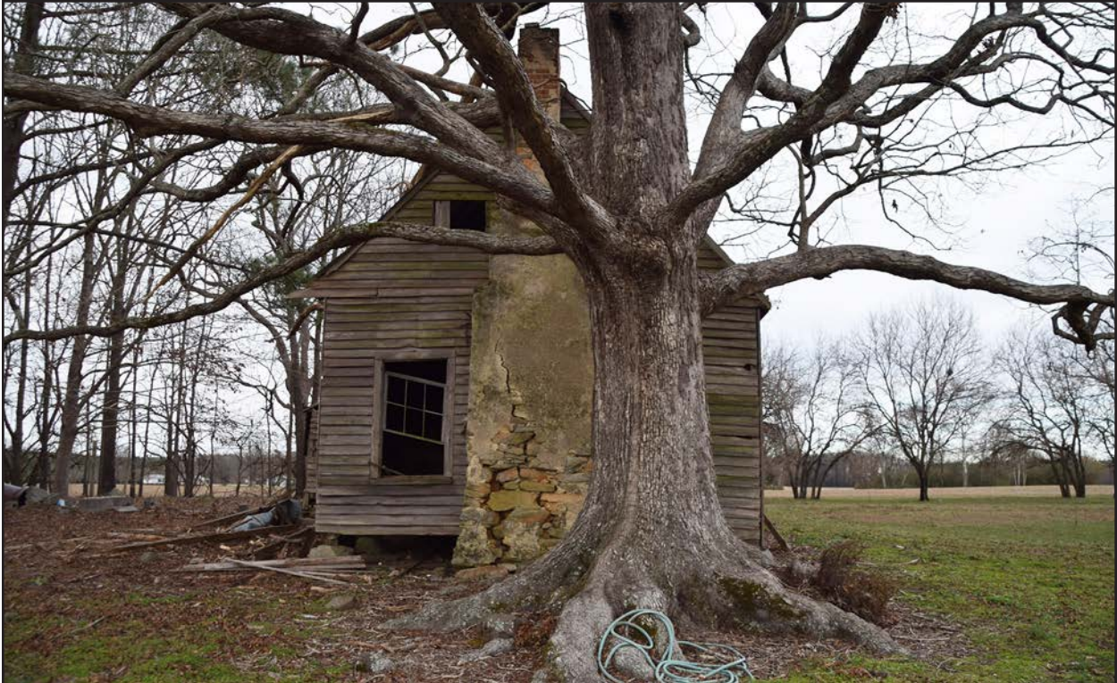
Photo 132. NS0650, cabin, facing east.
