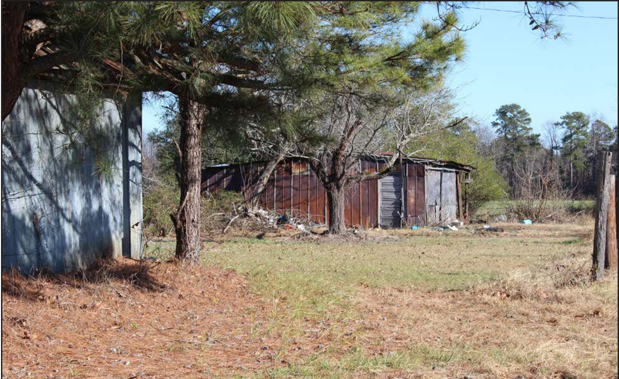
Photo 70. JT0957, gabled accessory structure 3, facing east.
