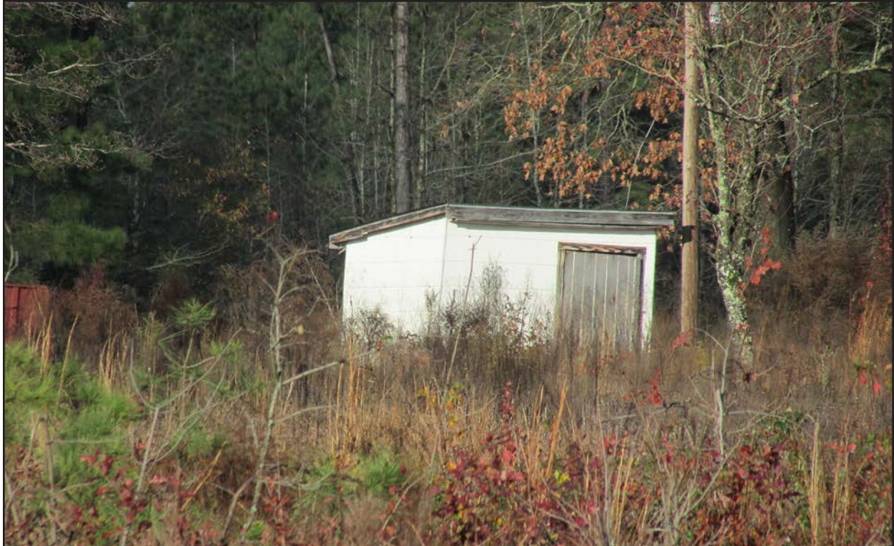
Photo 170. RB0678, well house, facing north.
