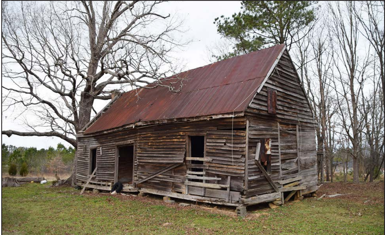
Photo 130. NS0650, cabin, facing northwest.
