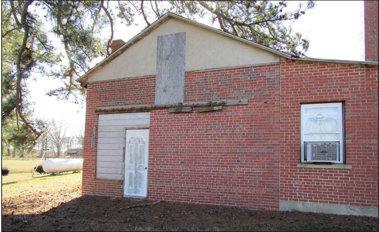
Photo 19. HX0021, barn door on smokehouse, facing south.
