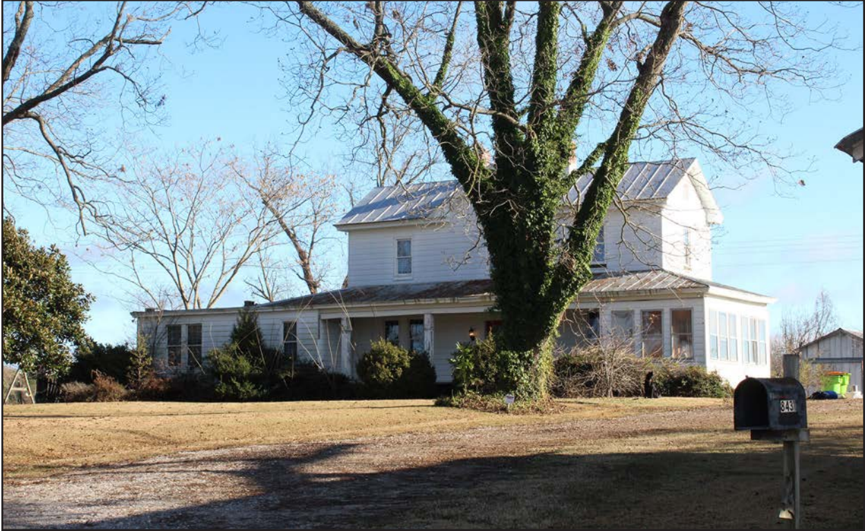
Photo 27. HX0227, main house, facing northeast.
