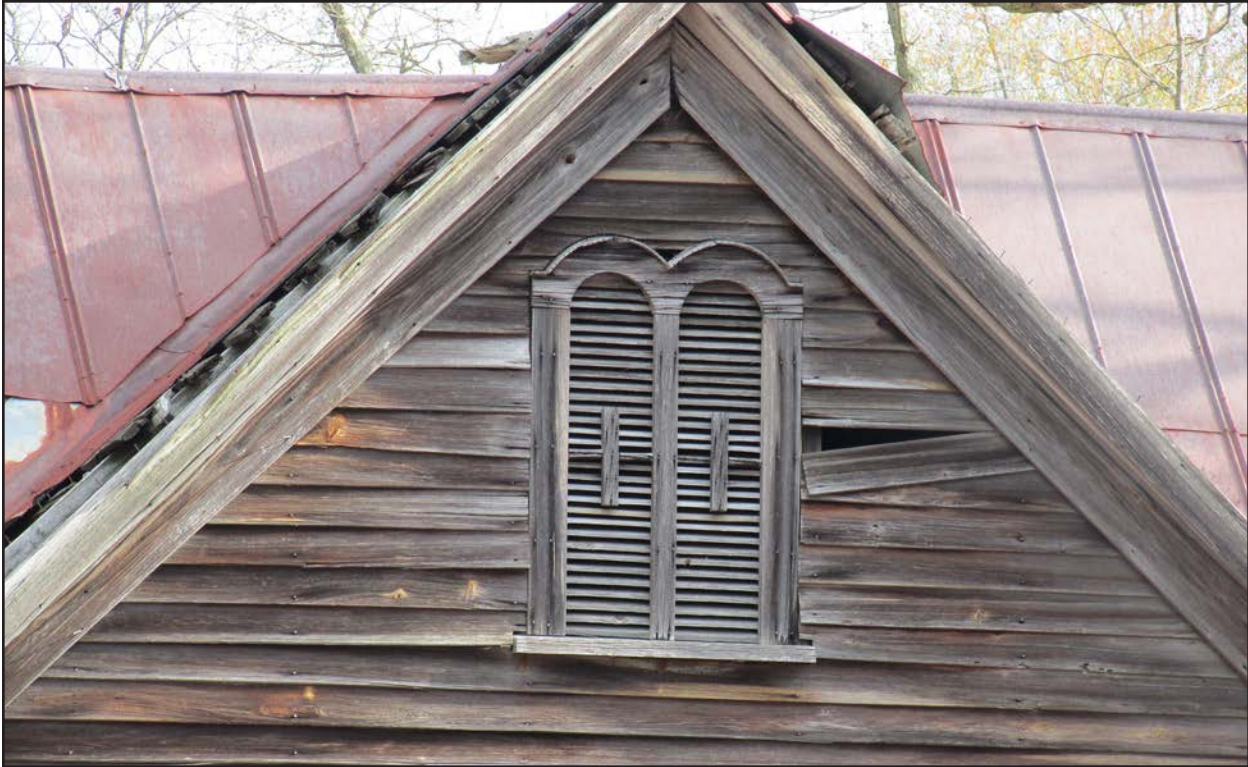
Photo 114. JT1937, vent details, facing east.
