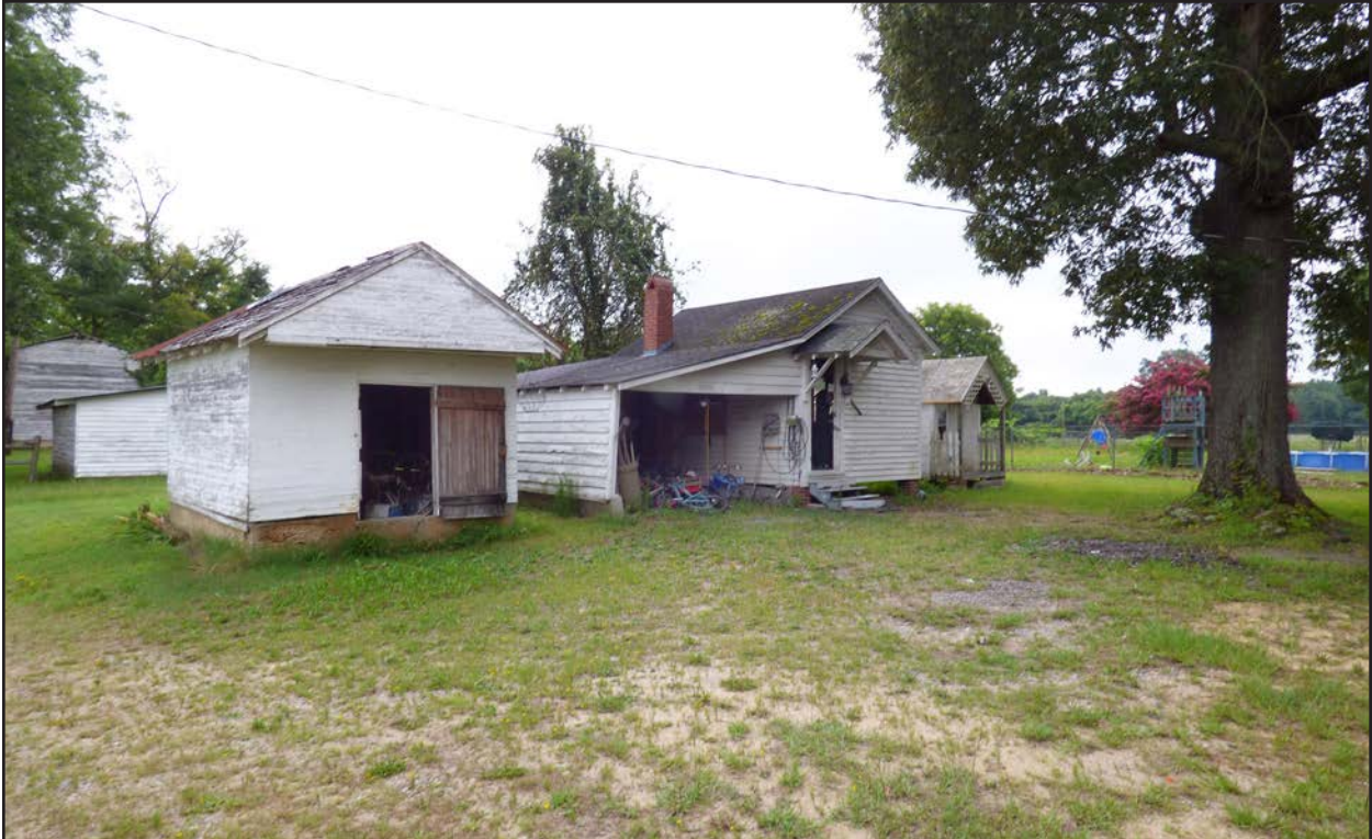
Photo 146. NS1493, well house, summer kitchen, meat shed, facing northeast.
