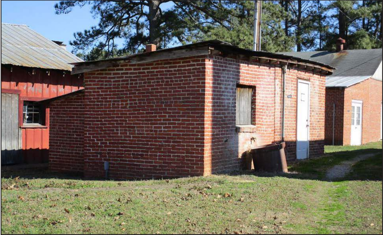
Photo 21. HX0021, pumphouse, facing east.
