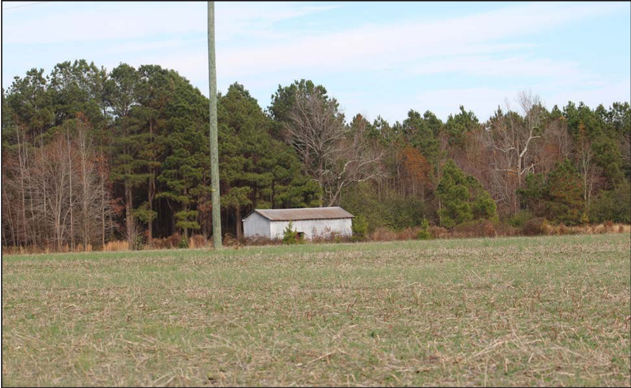
Photo 86. JT1913, storage structure, facing northeast.
