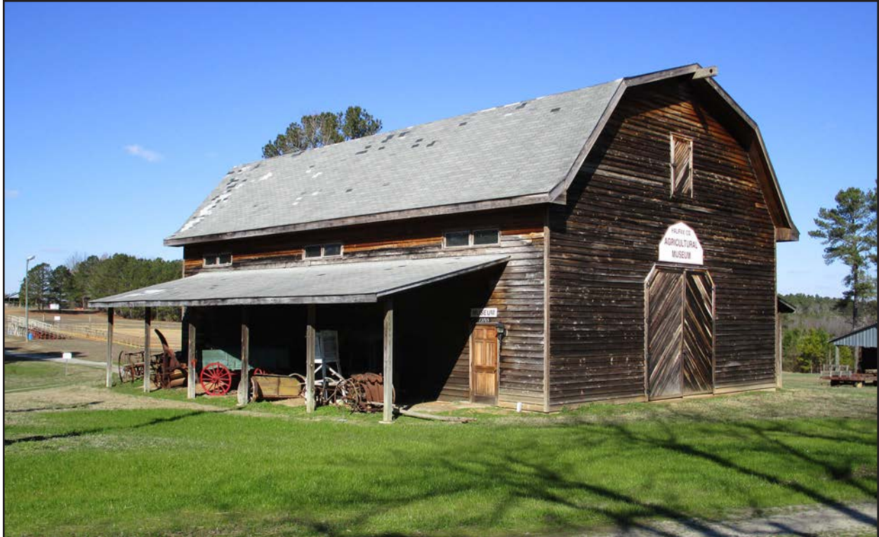
Photo 10. HX0021, barn, facing north.
