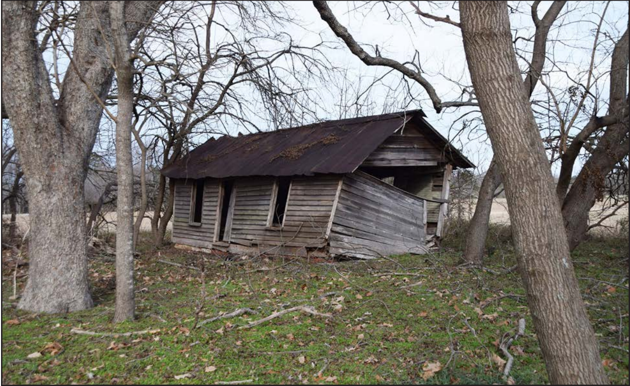
Photo 133. NS0650, summer kitchen, facing northeast
