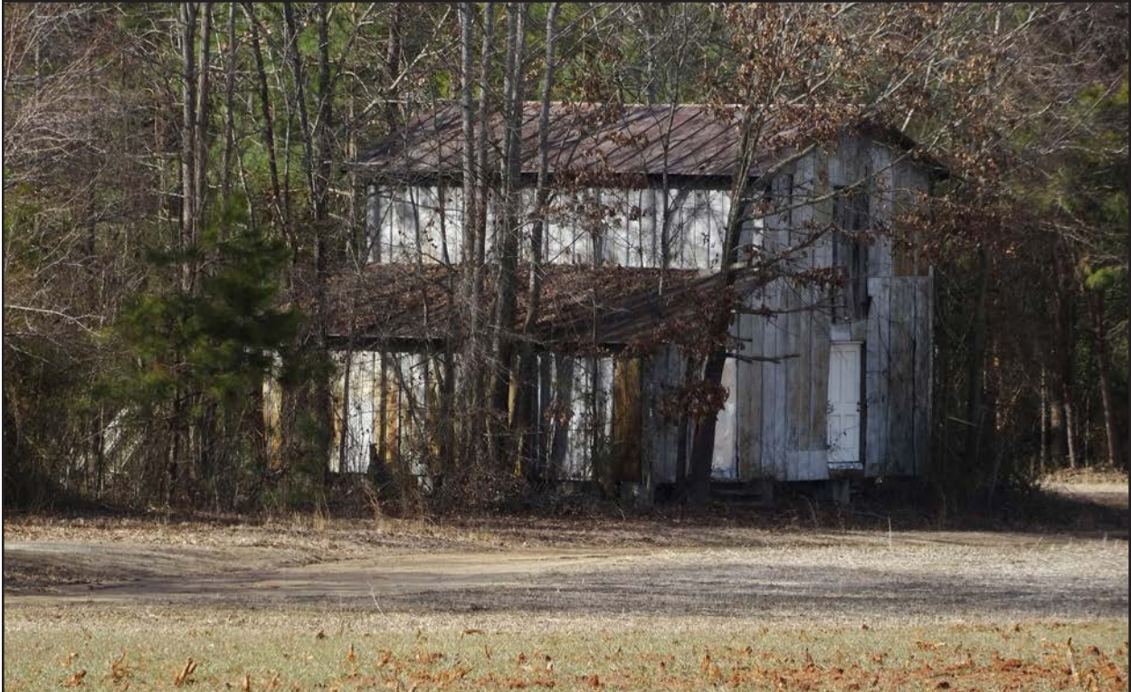
Photo 178. WL2002, barn, facing north-northwest.
