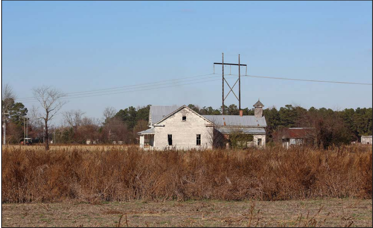
Photo 121. JT1969, facing north.
