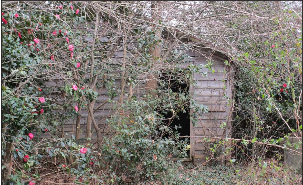
Photo 110. JT1935 accessory structure 2, facing south.
