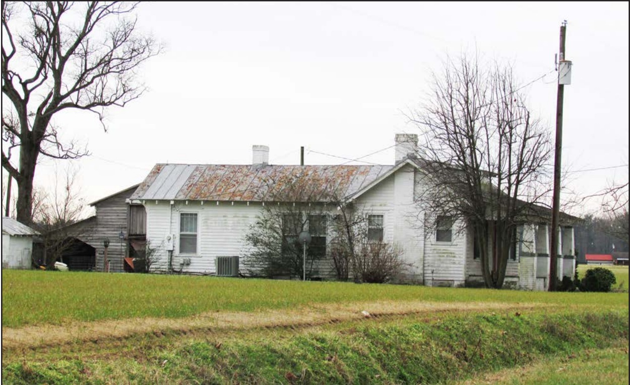
Photo 162. NS1517, dwelling, facing southwest.
