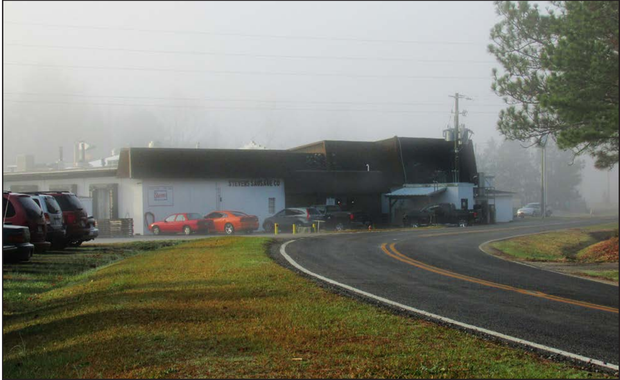
Photo 95. JT1921 (Stevens Sausage Company plant), facing south.
