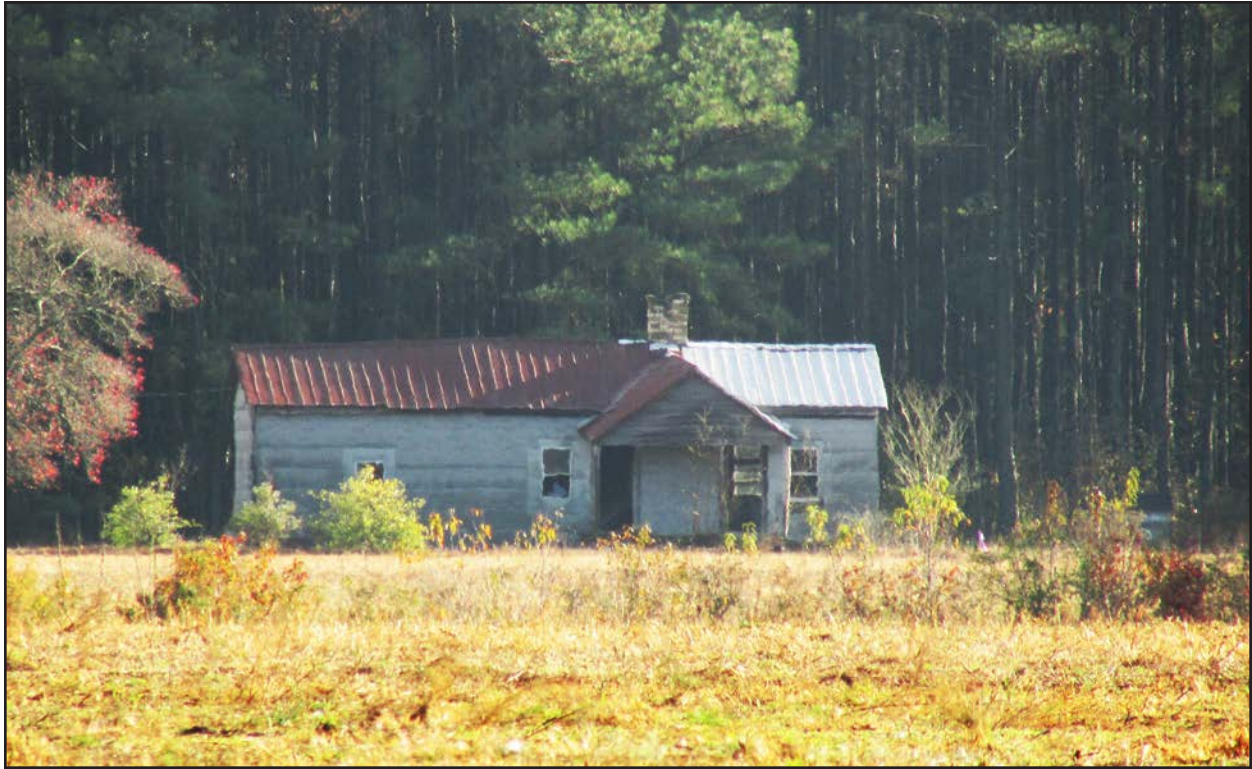
Photo 171. RB0680, house, facing southeast.
