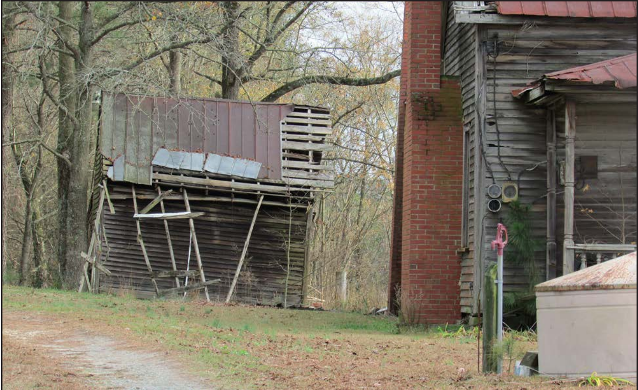
Photo 116. JT1937, accessory structure facing east.
