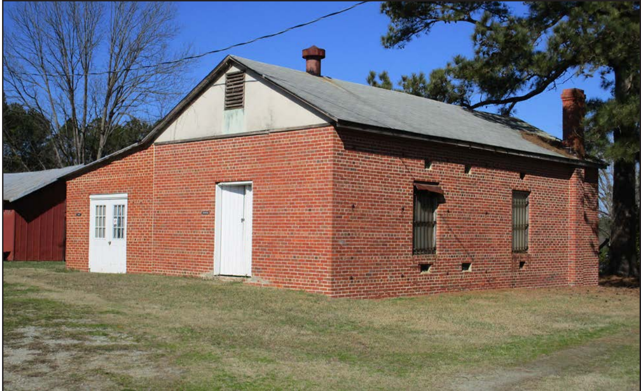
Photo 18. HX0021, smokehouse, facing north.
