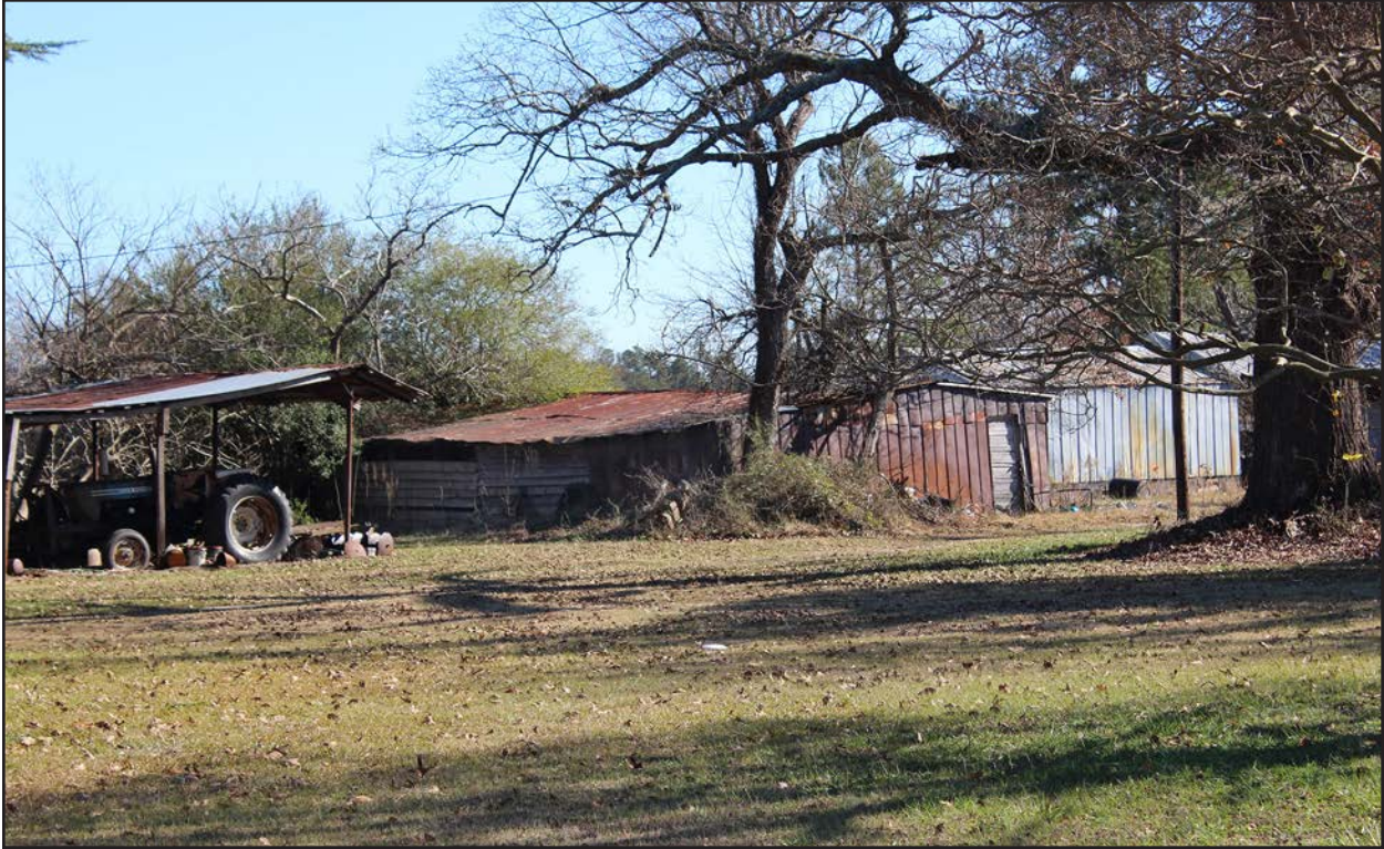
Photo 69. JT0957, gabled accessory structure 3, facing southeast.
