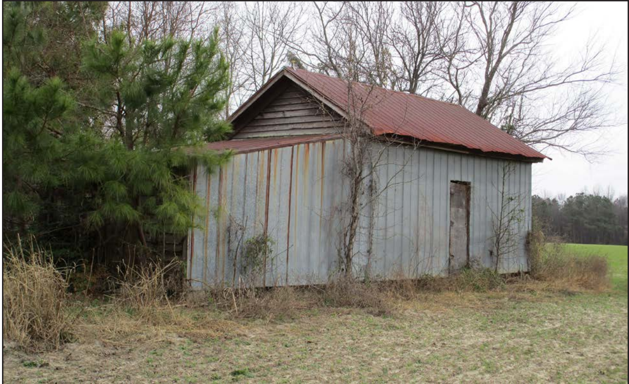
Photo 106. JT1935 accessory structure 1, facing southeast.
