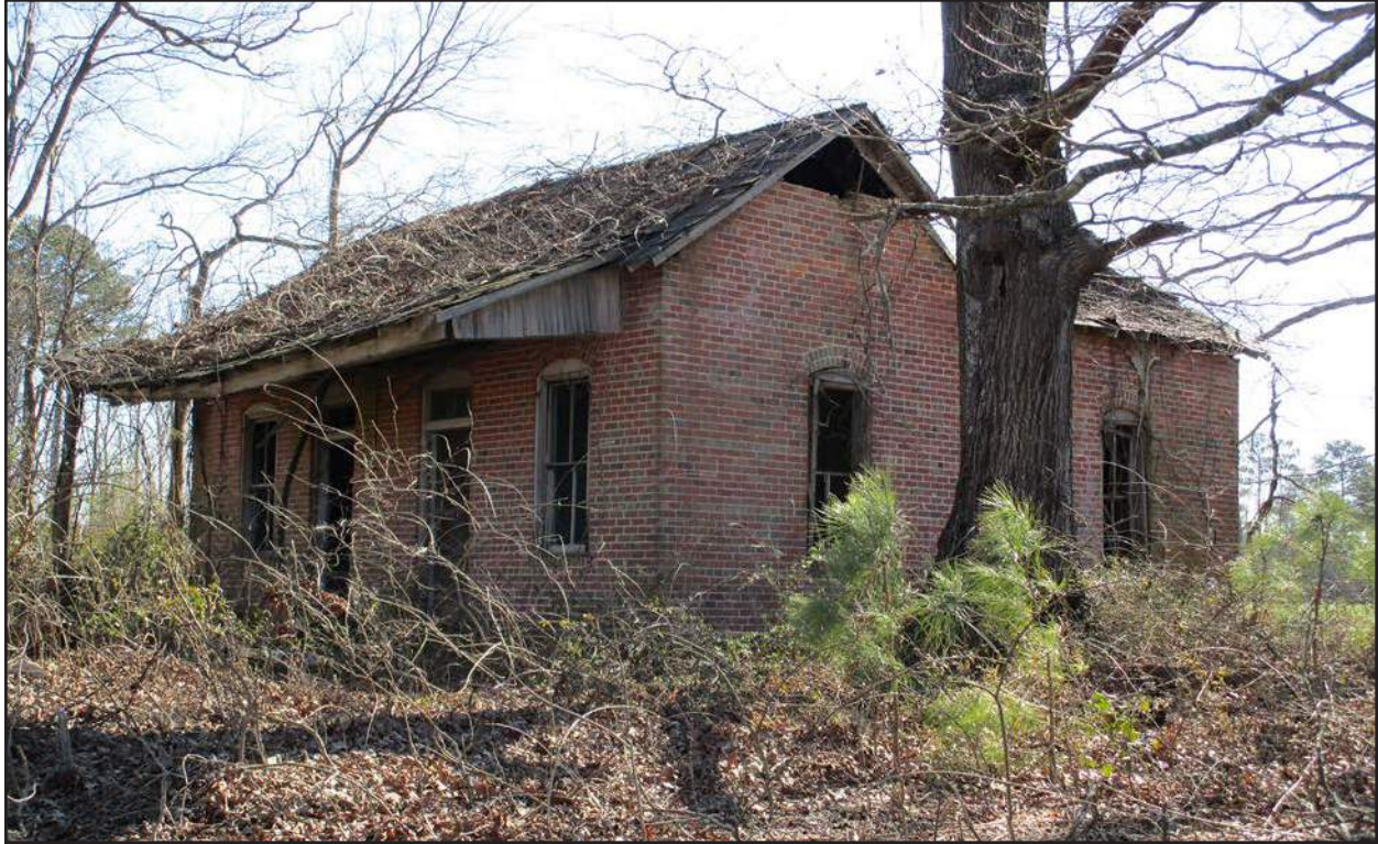
Photo 39. HX0354, facing south.
