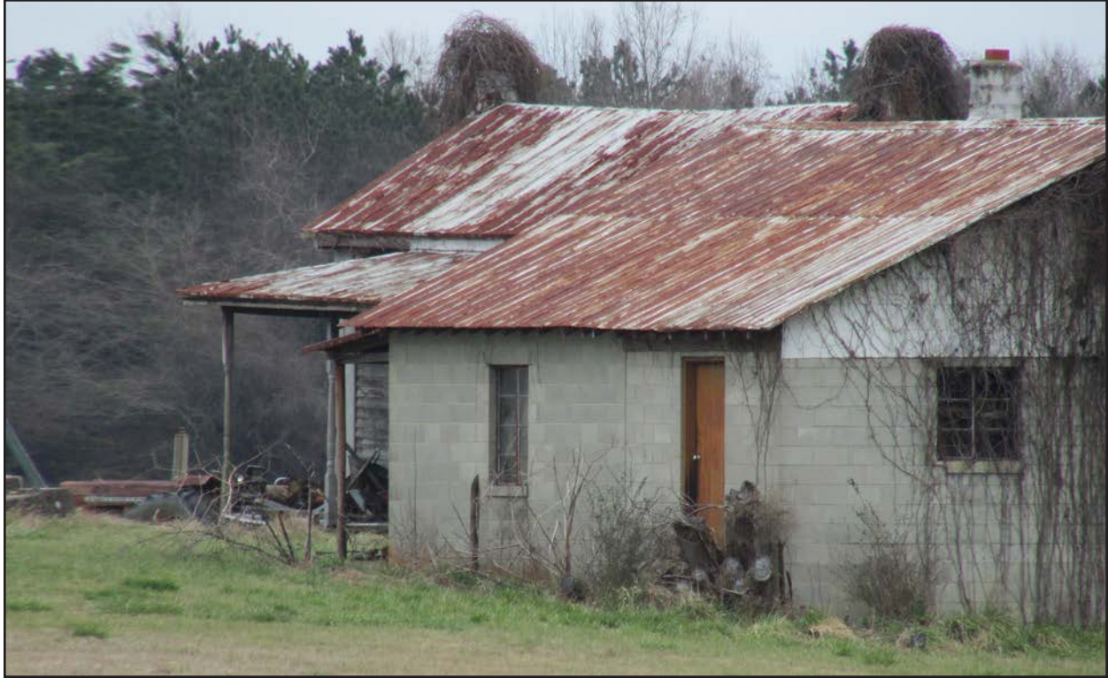
Photo 149. NS1504, facing northeast.
