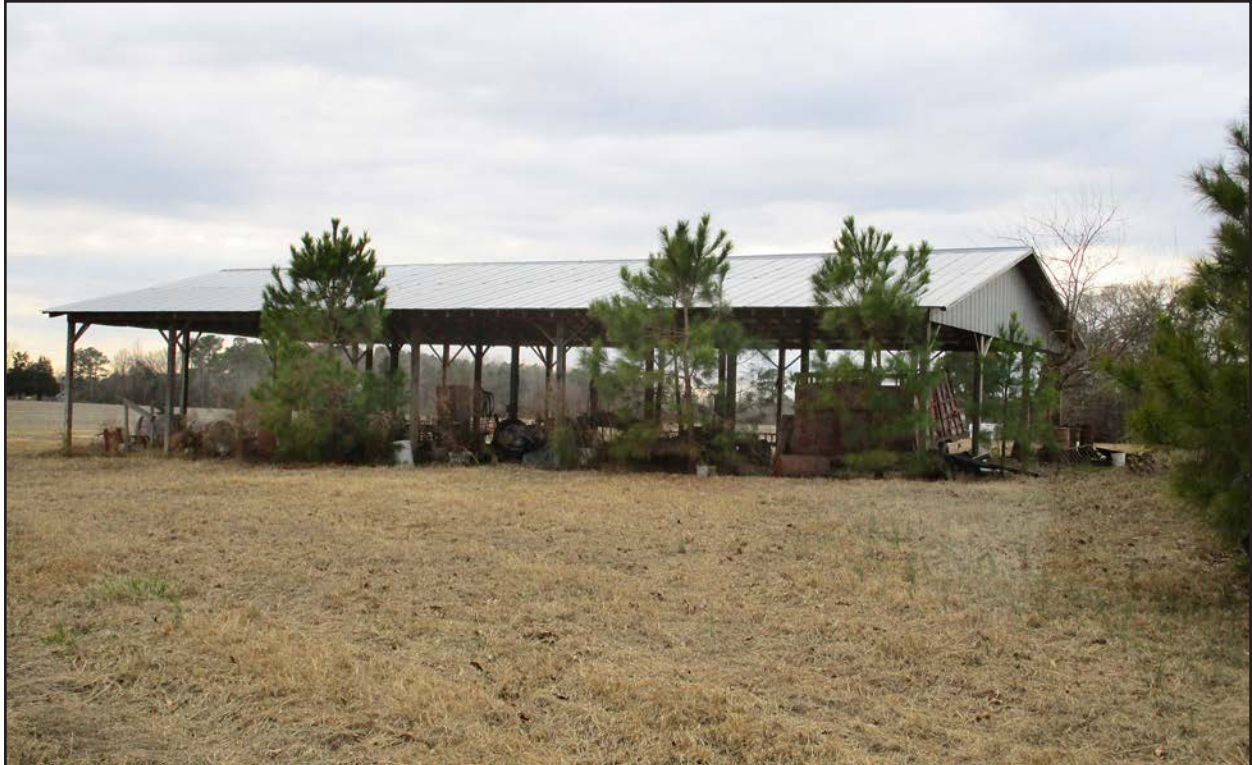
Photo 160. NS1508, pole shed, facing southwest.
