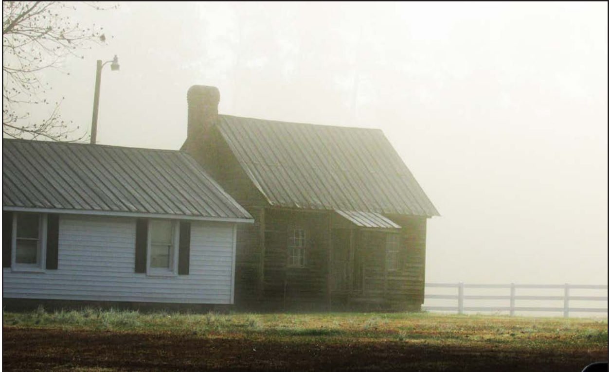
Photo 92. JT1920, log cabin, facing southeast.
