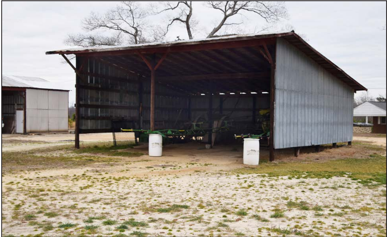
Photo 49. HX1581, equipment shelter, facing northeast.
