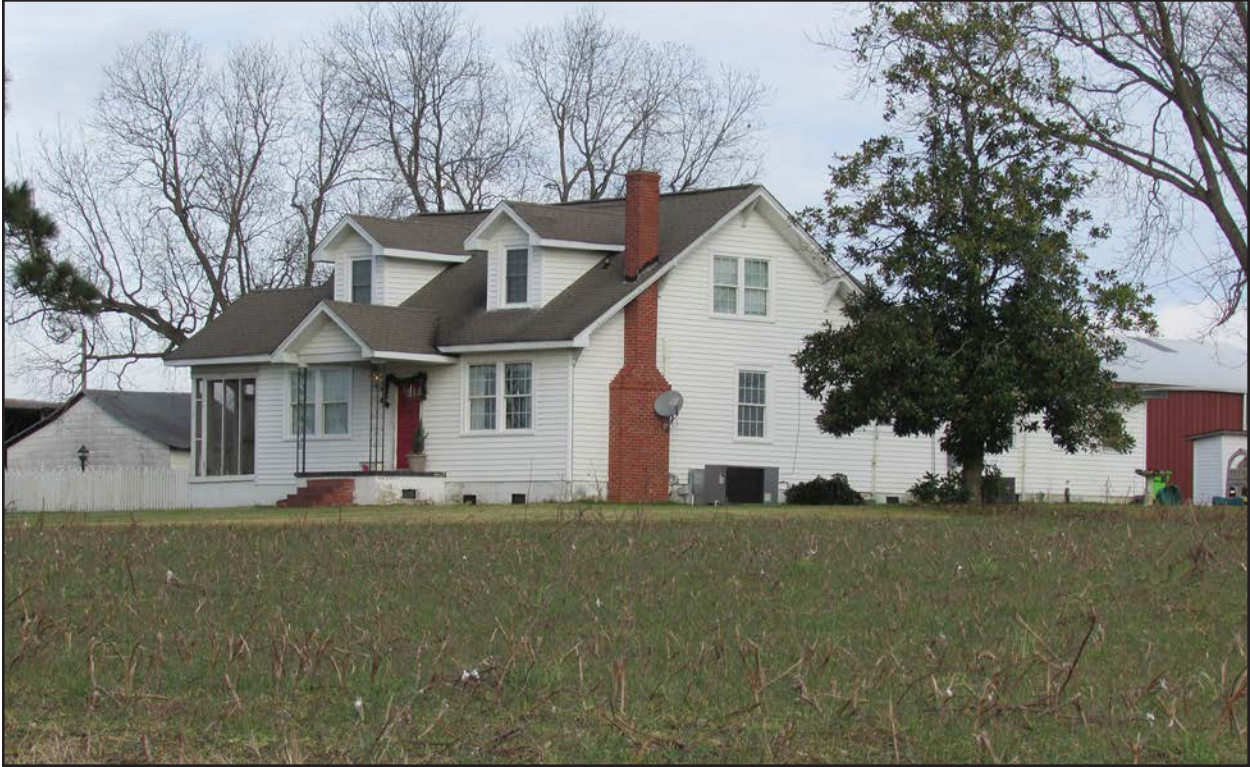
Photo 53. HX1583, facing northeast.
