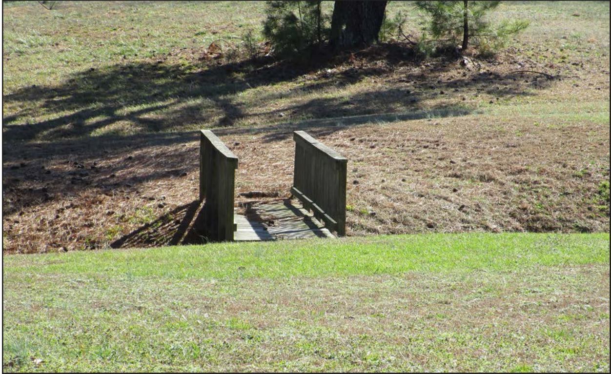
Photo 25. HX0021, wooden bridge, facing south-southeast.
