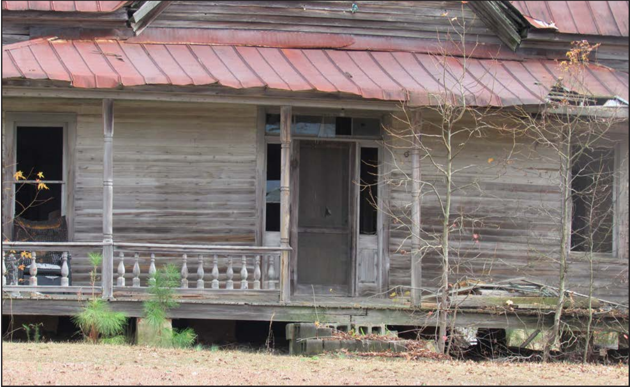
Photo 115. JT1937, main entrance facing east.
