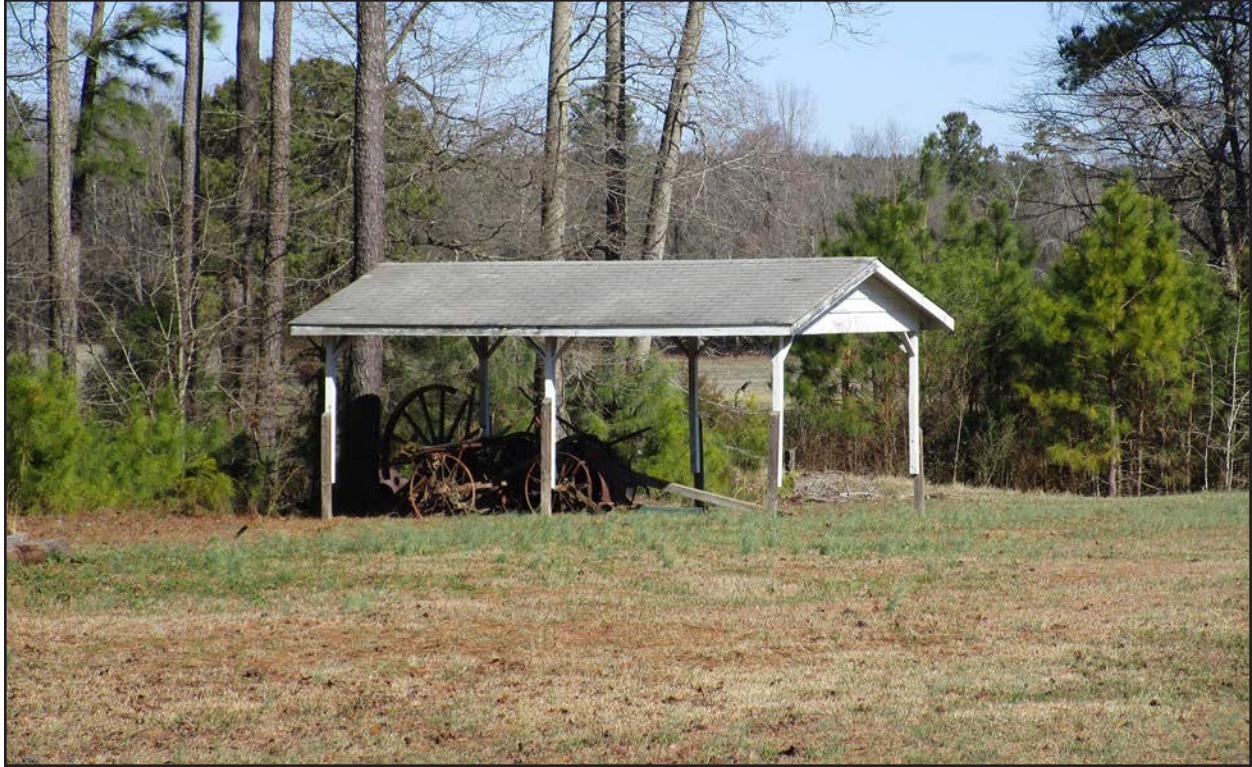
Photo 11. HX0021, shed, facing north-northeast.
