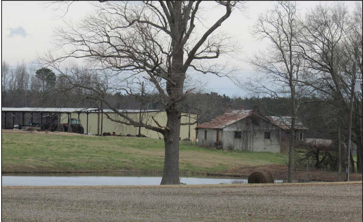
Photo 148. NS1504, facing northeast.
