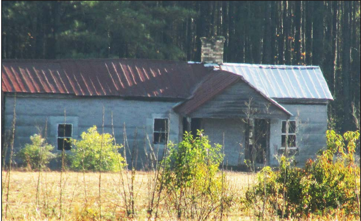
Photo 172. RB0680, house, porch detail.
