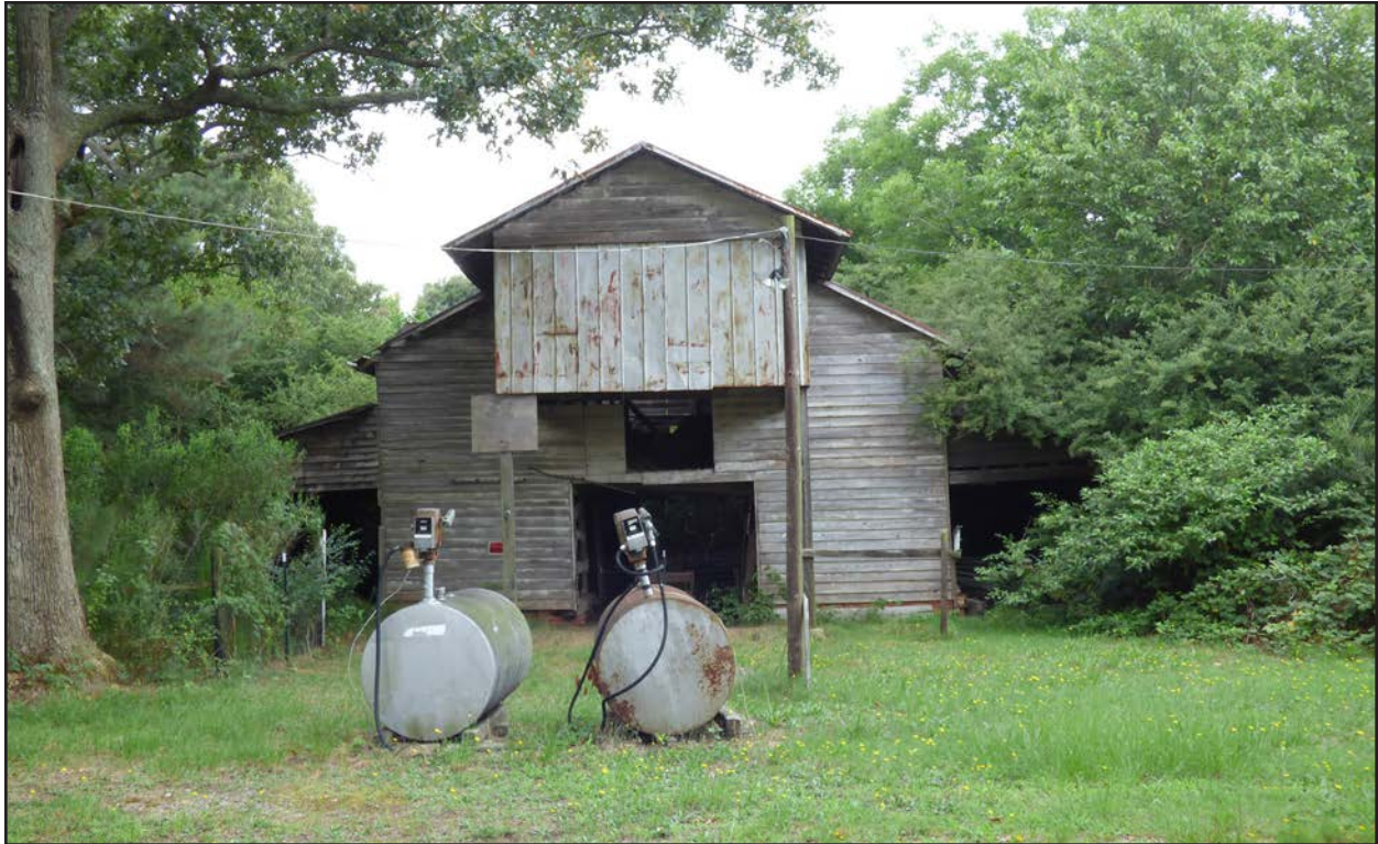
Photo 139. NS1493, hay barn, facing west.
