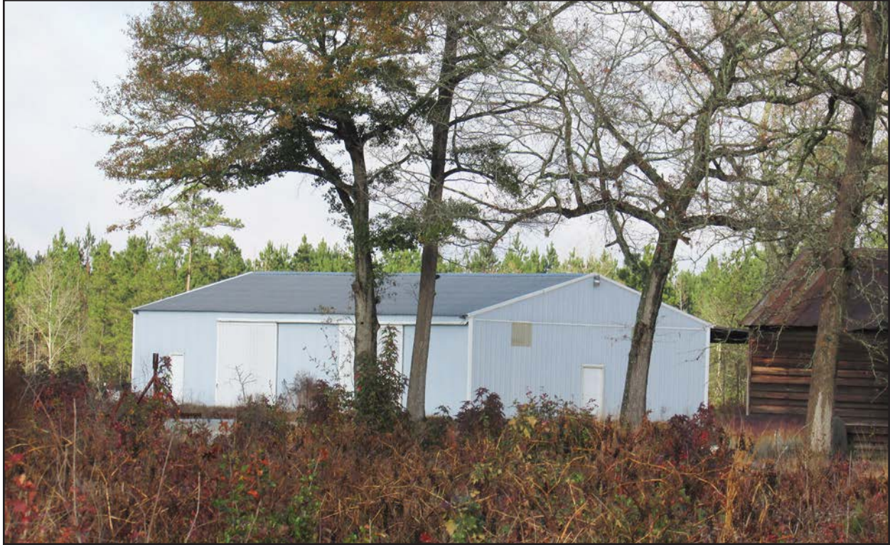
Photo 169. RB0678, agricultural/storage outbuilding, facing north.
