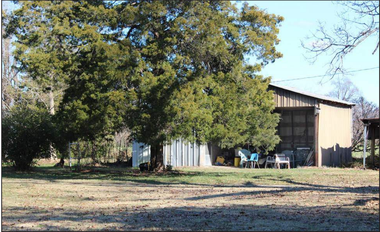
Photo 67. JT0957, storage structure, facing east-northeast.
