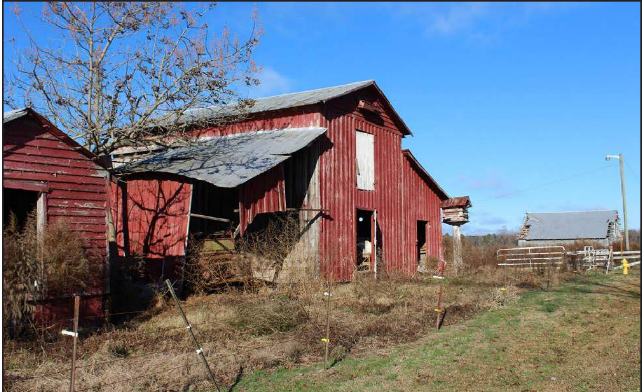
Photo 36. HX0229, facing north-northwest.
