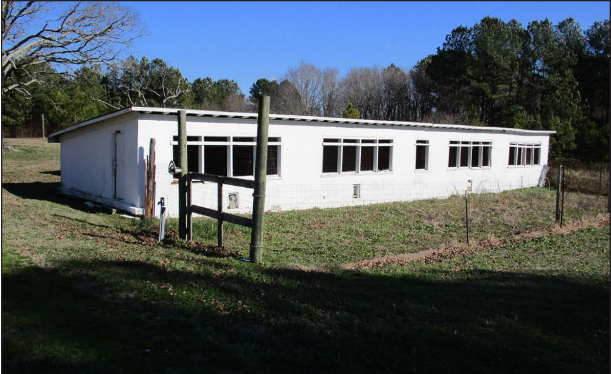
Photo 16. HX0021, chicken house, facing east.
