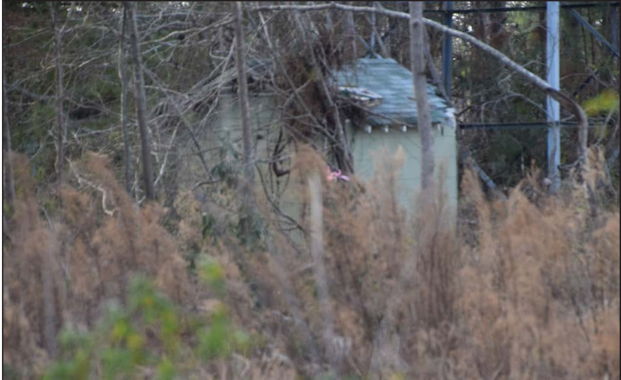
Photo 76. JT1860 (Smithfield Fire Lookout Tower), outbuilding, facing west-northwest.
