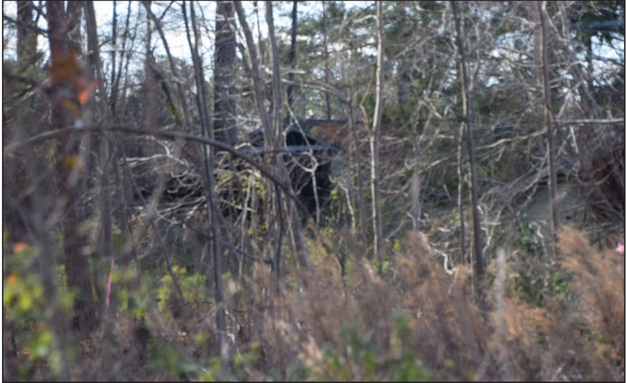
Photo 77. JT1860 (Smithfield Fire Lookout Tower), equipment shed facing northwest.
