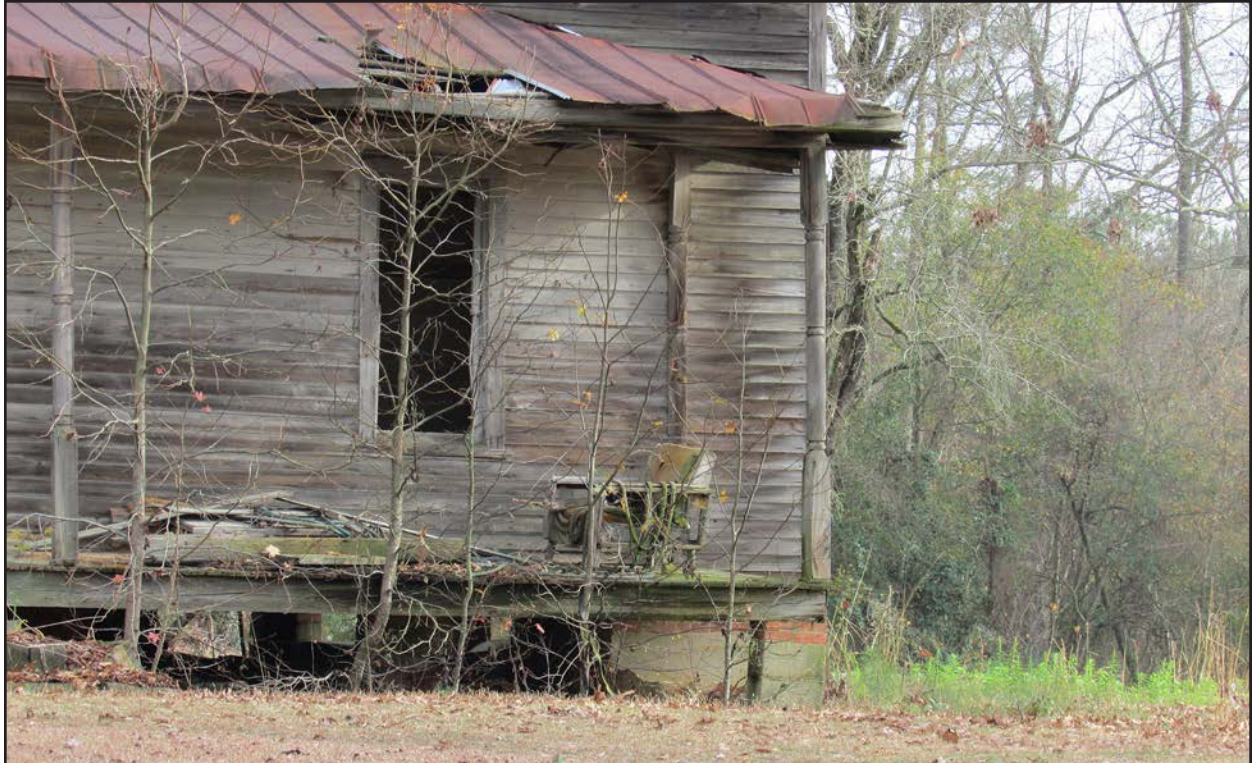
Photo 112. JT1937, foundation, facing southeast.
