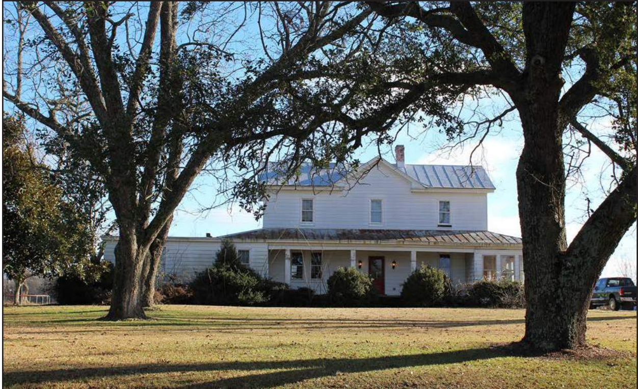
Photo 26. HX0227, main house, facing east.
