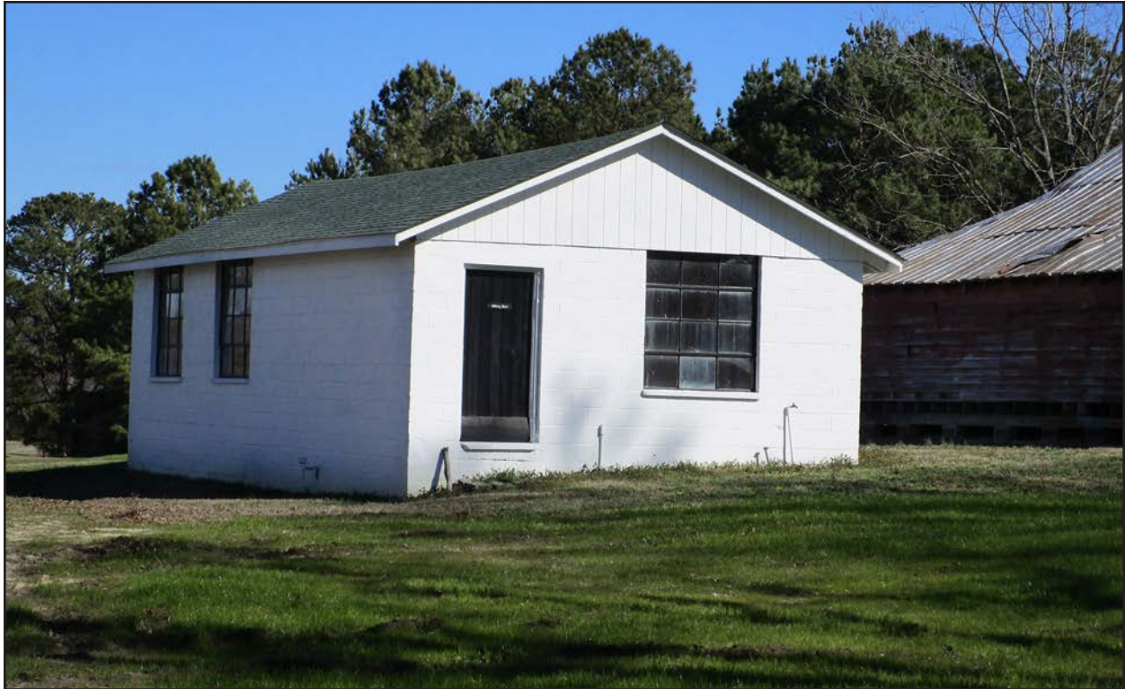
Photo 13. HX0021, milking barn, facing northeast.
