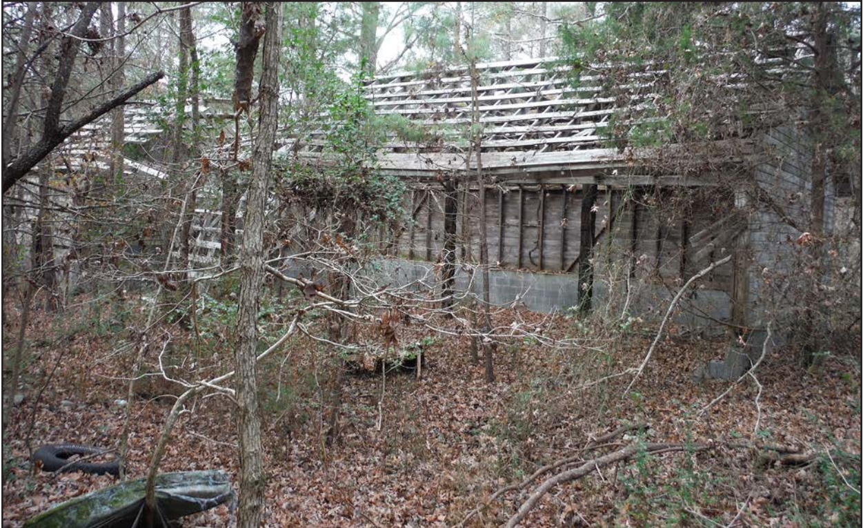
Photo 58. HX1597, barn, facing north.
