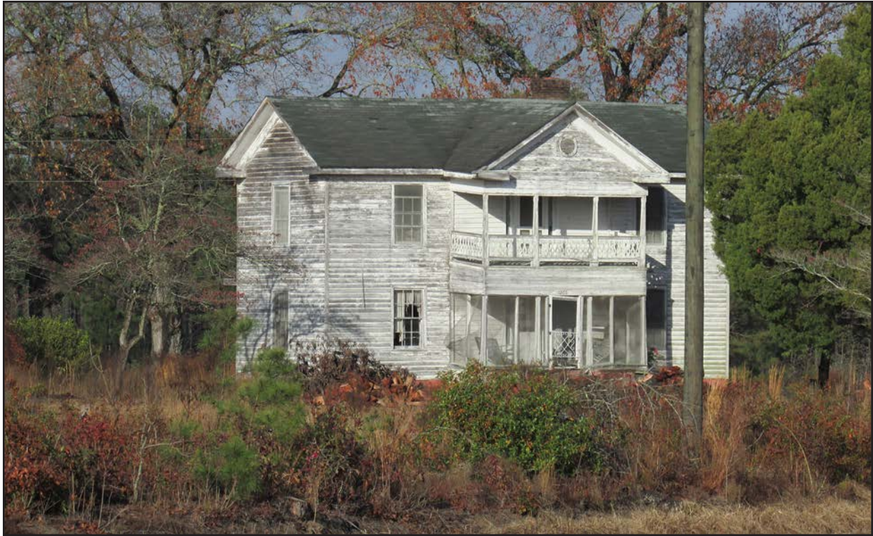
Photo 165. RB0678, house, facing northwest.
