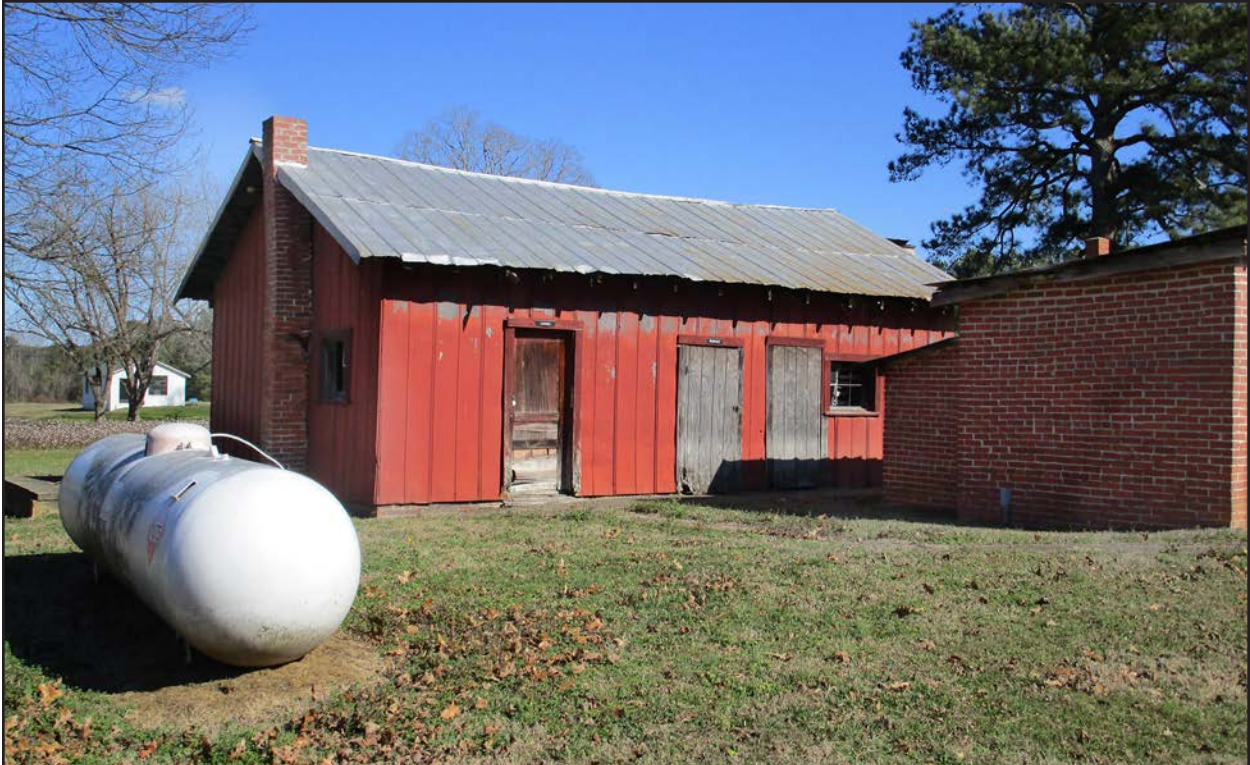
Photo 22. HX0021, wash room/laundry, facing northeast.
