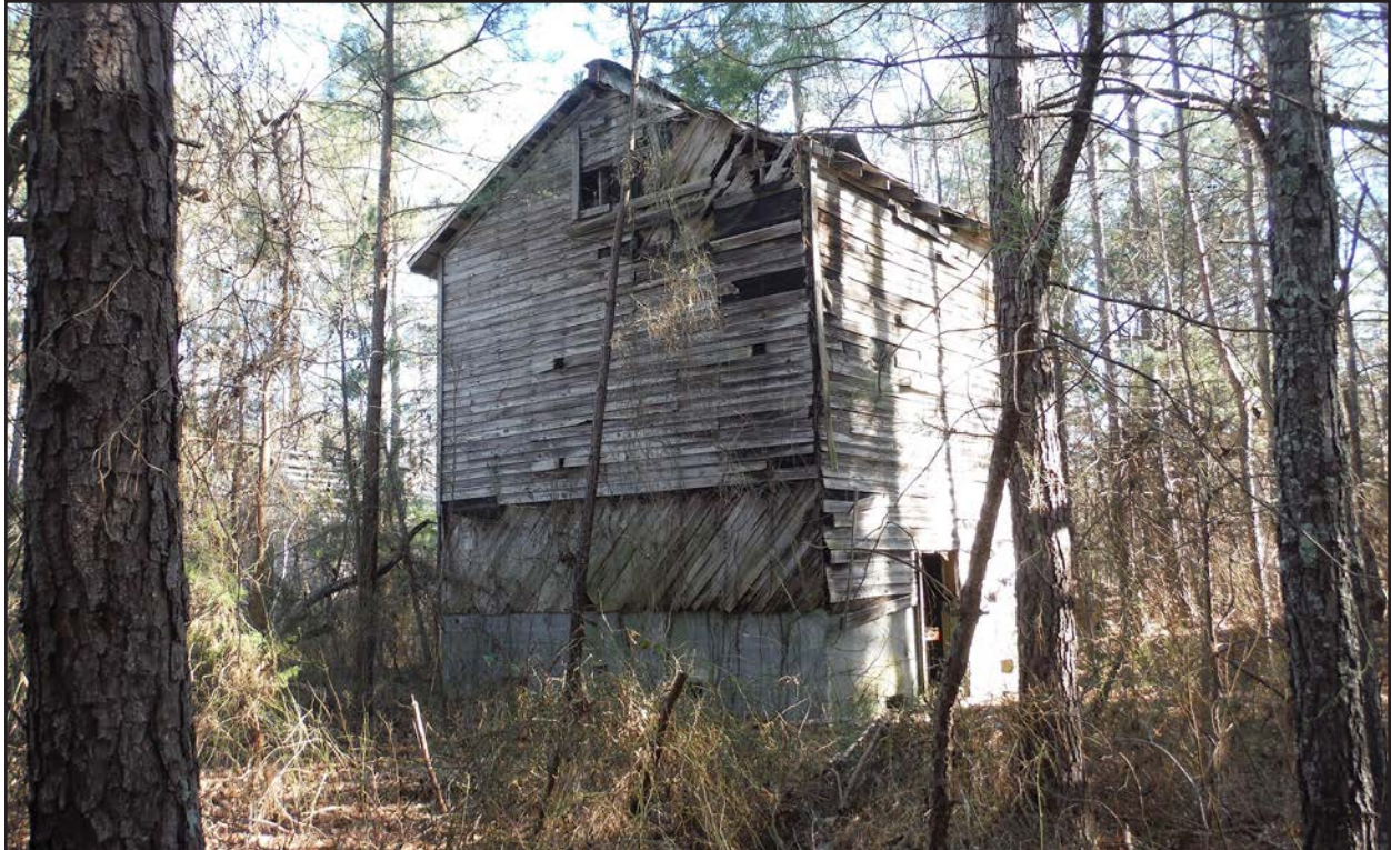
Photo 60. HX1597, tobacco barn 2, facing northeast.
