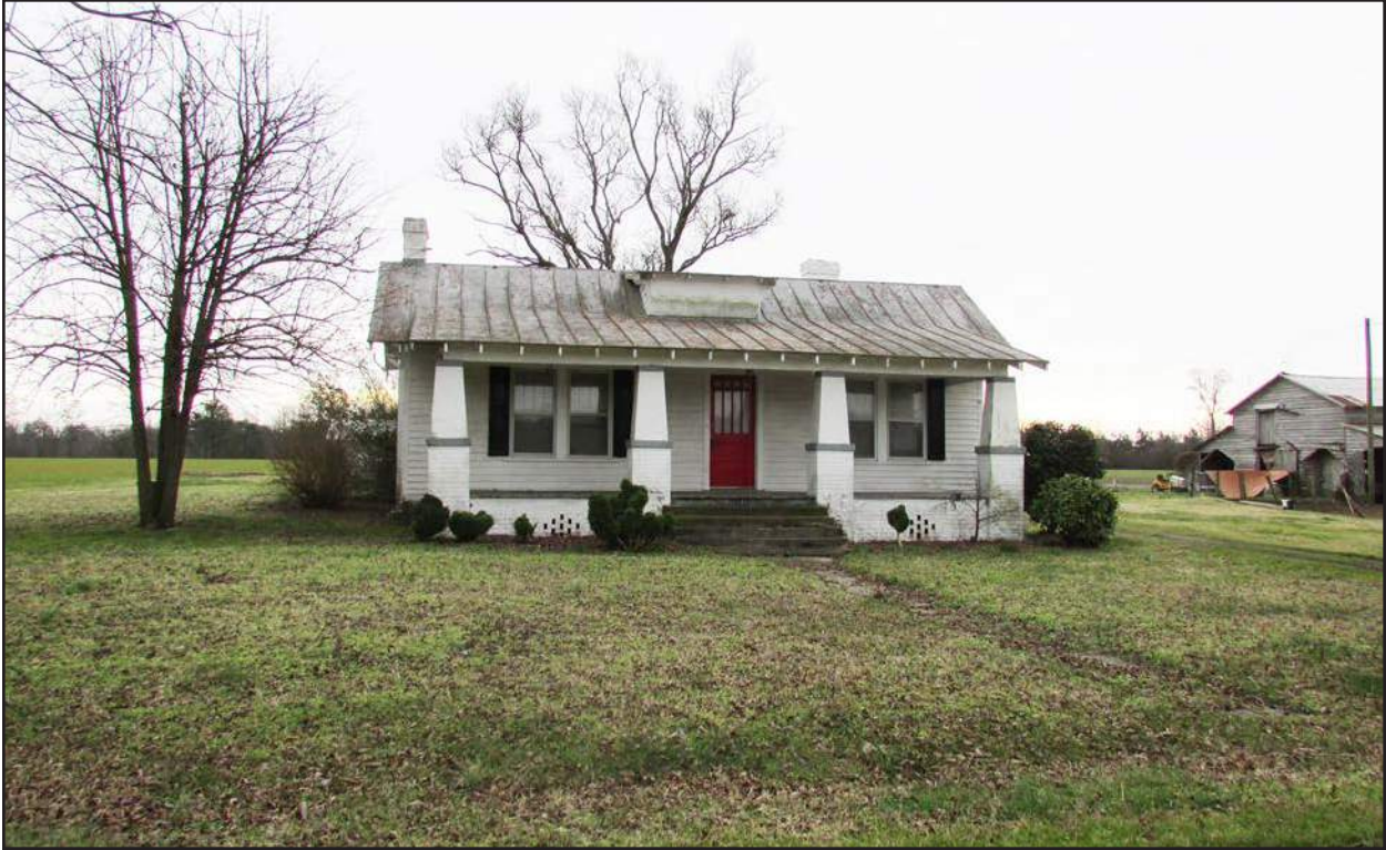
Photo 161. NS1517, dwelling, facing south-southeast.
