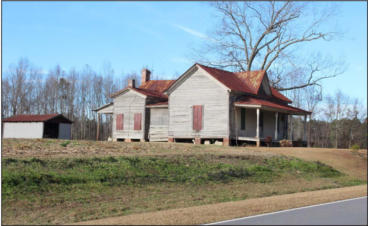
Photo 181. WL2012, facing north-northwest.
