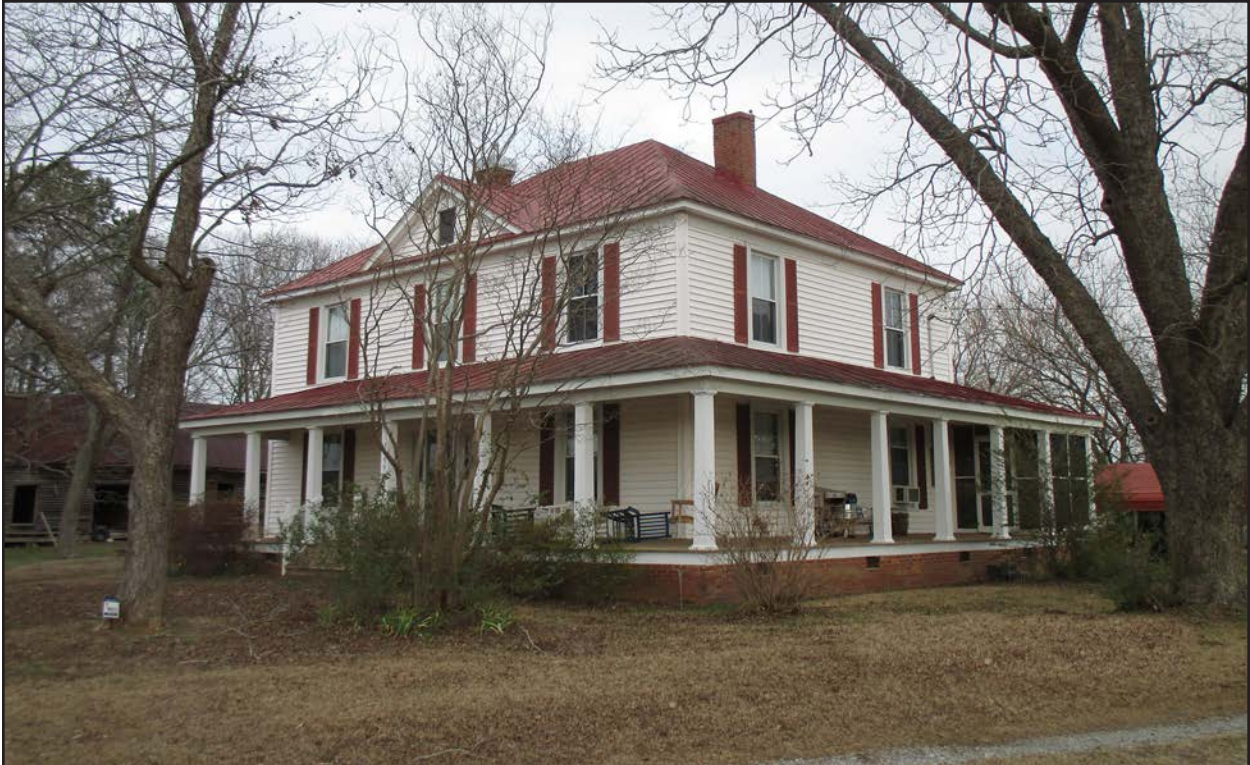
Photo 124. NS0650, house, facing northeast.
