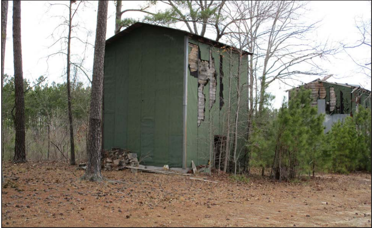
Photo 153. NS1508, ca. 1950–1960s storage structure, facing northwest.
