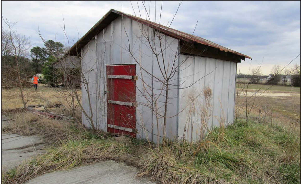
Photo 158. NS1508, ca. 1960 structure, facing southwest.
