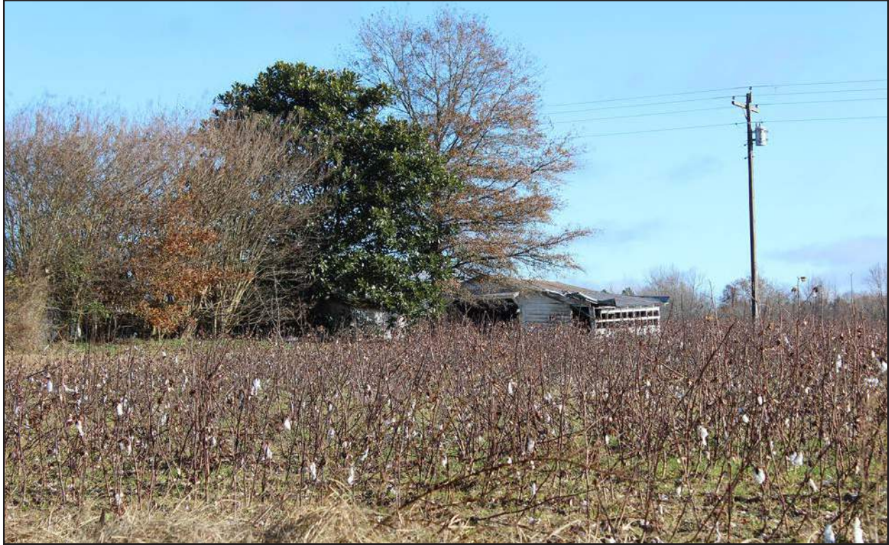
Photo 31. HX0227, rear accessory structure, facing northeast.
