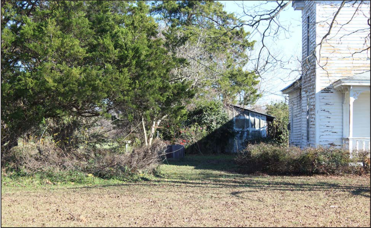
Photo 65. JT0957, gabled accessory structure 1, facing east.
