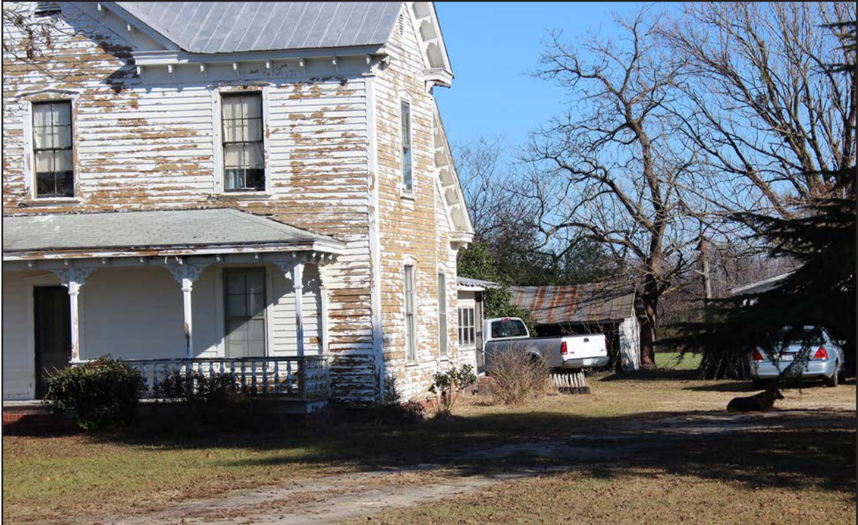
Photo 66. JT0957, gabled accessory structure 2, facing east-northeast.
