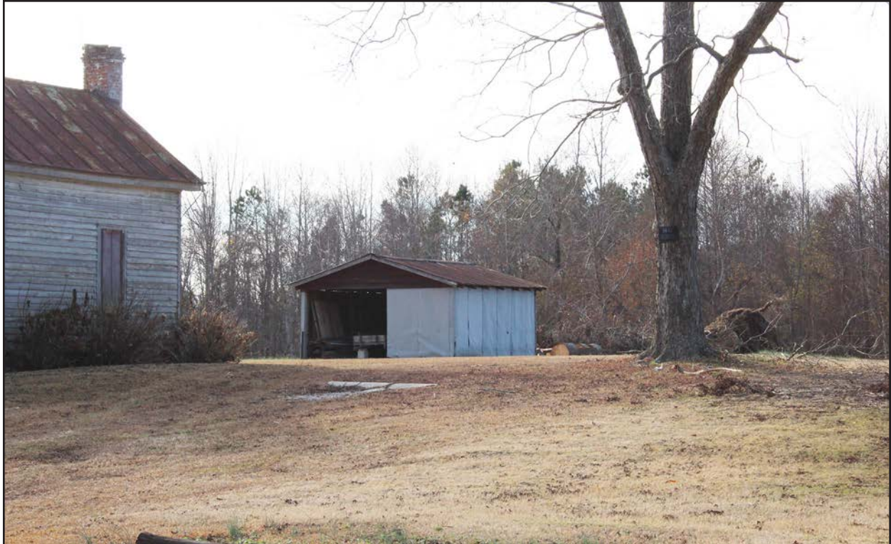
Photo 182. WL2012, outbuilding, facing southwest.
