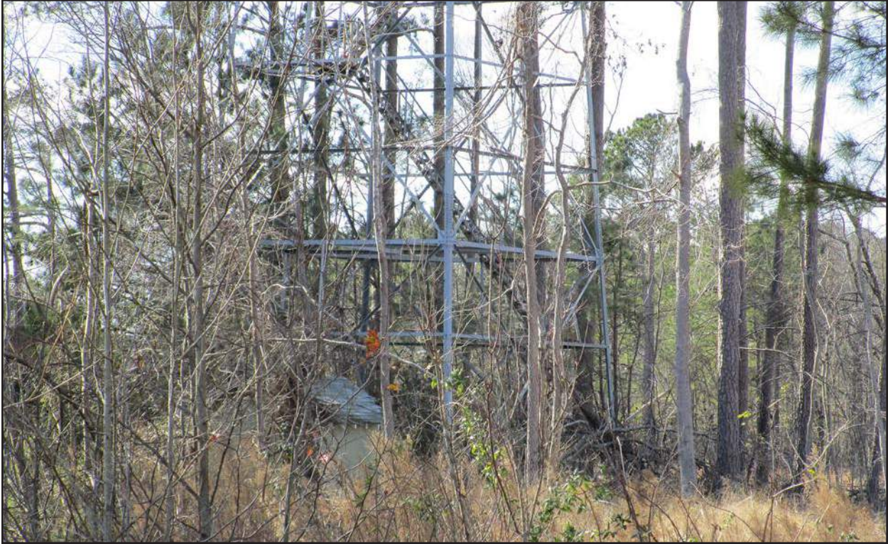
Photo 73. JT1860 (Smithfield Fire Lookout Tower), fire tower base, facing northwest.
