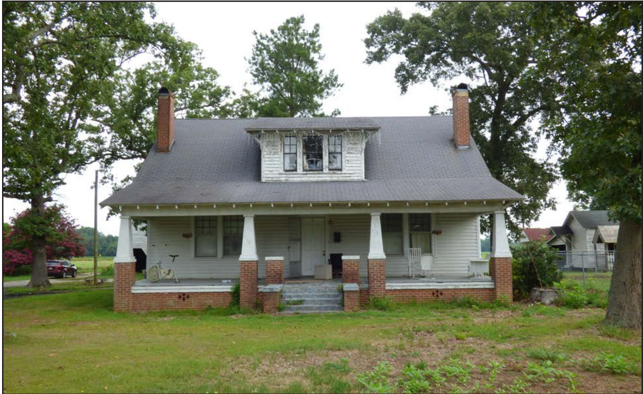
Photo 137. NS1493, dwelling, facing north.
