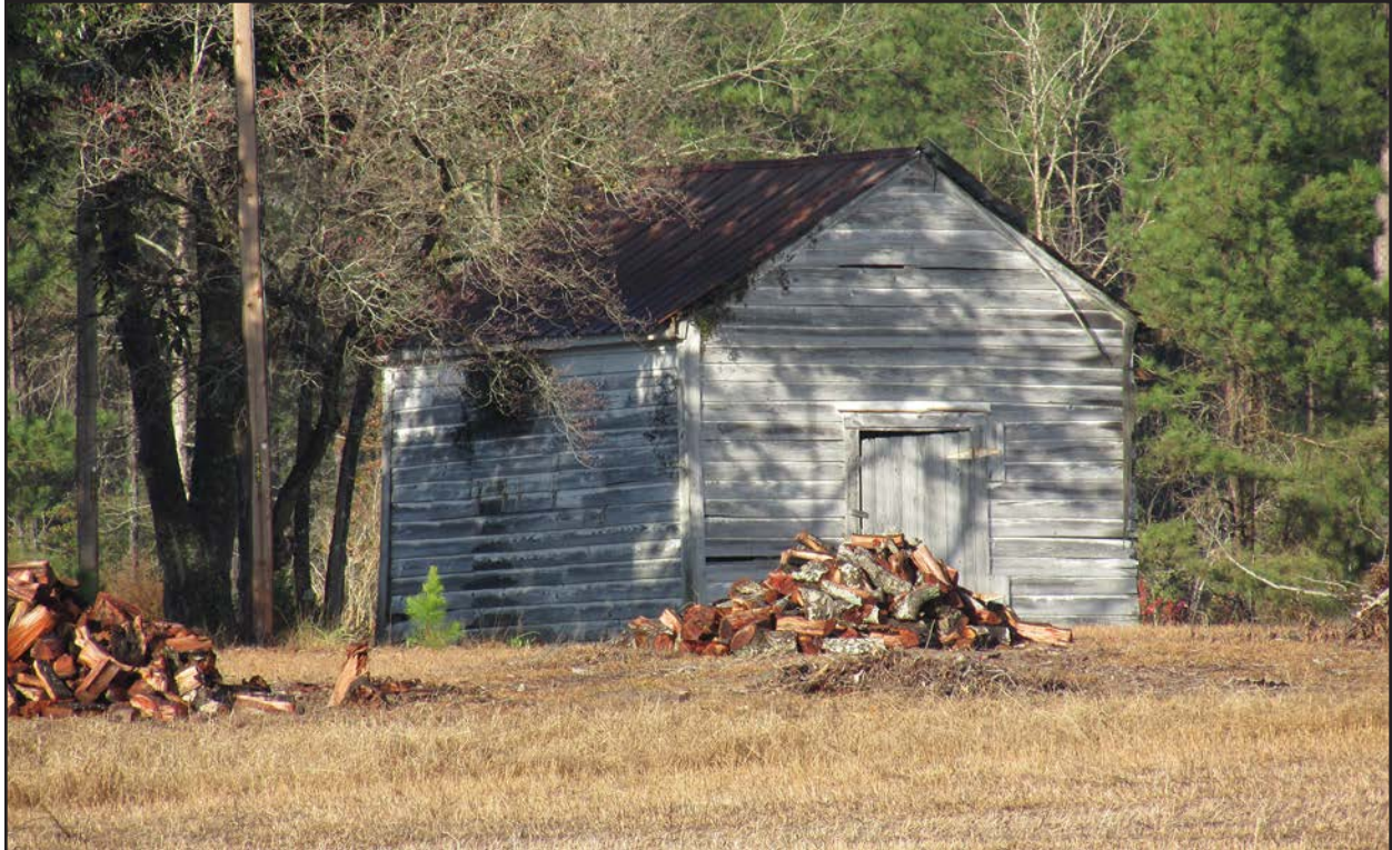
Photo 166. RB0678, shed, facing north.
