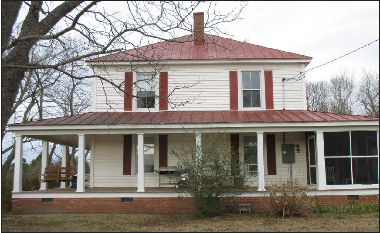
Photo 125. NS0650, house, facing north.
