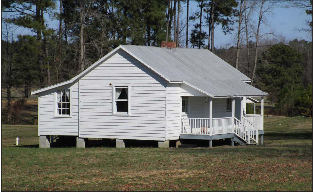
Photo 9. HX0021, house, facing northeast.
