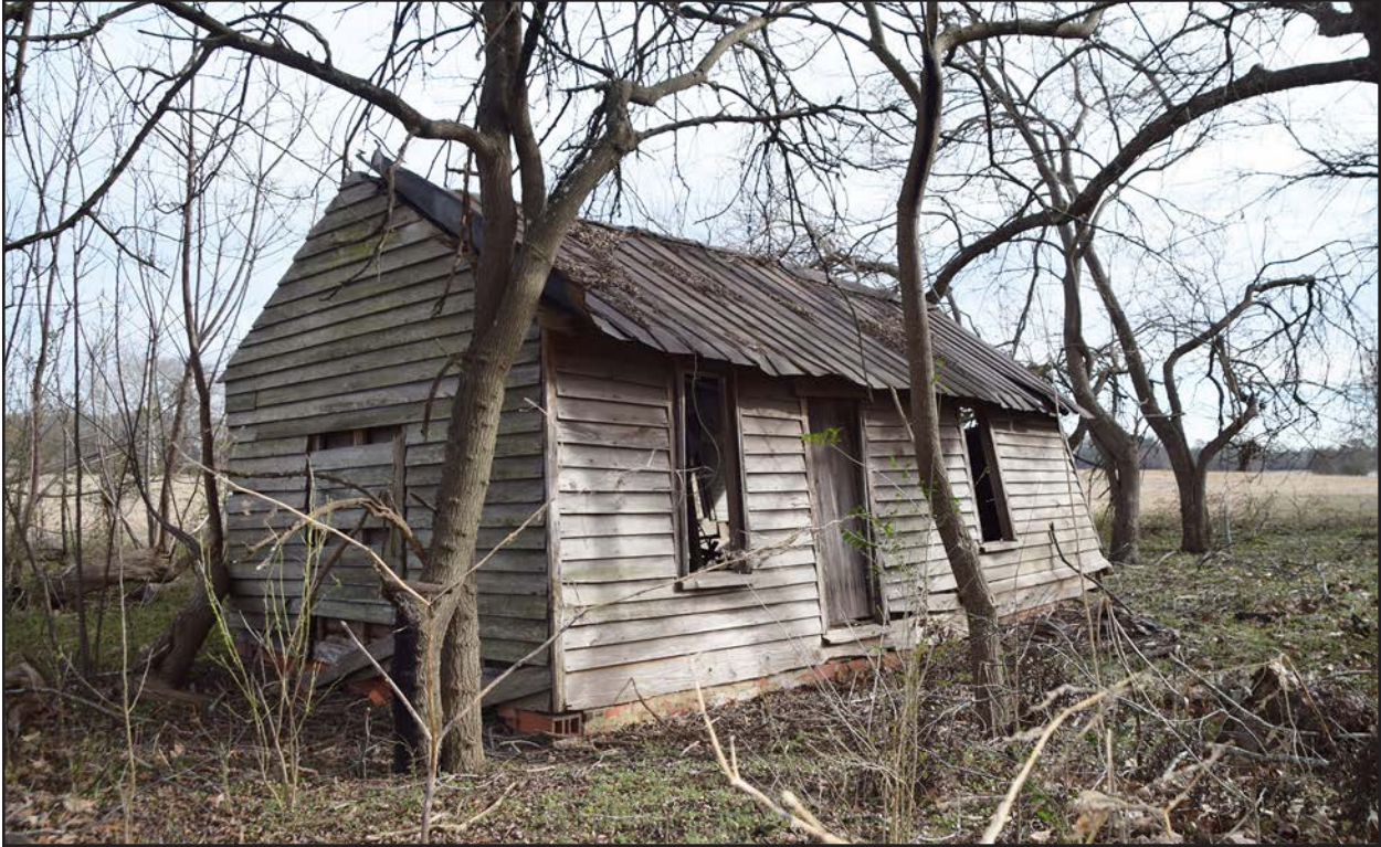
Photo 135. NS0650 summer kitchen, facing northeast.
